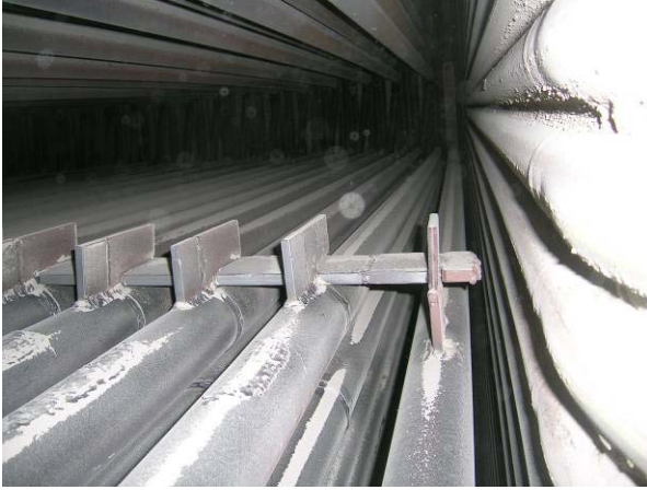
Figure 6. Secondary superheater tubes and supporting brackets. In this picture, the view is looking up words along the superheater tubes (lower left). The tubes on the right are part of the membrane wall.
