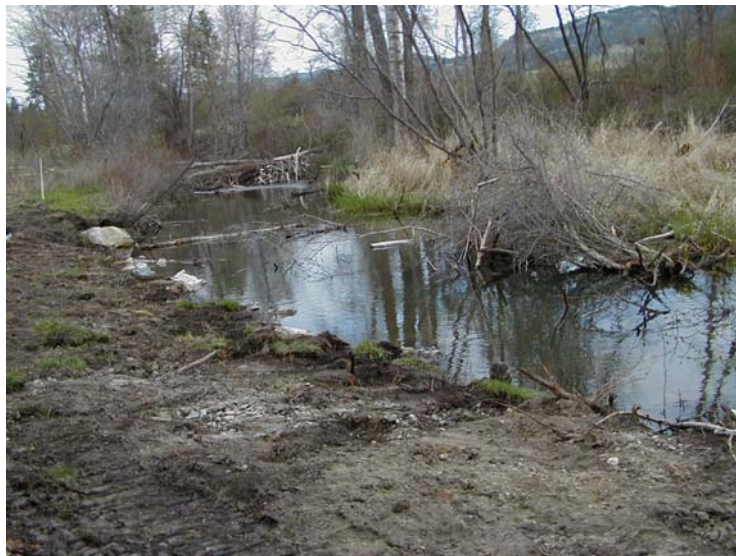
Figure 2: Bank of Dayton Creek after reshaping and armoring.
