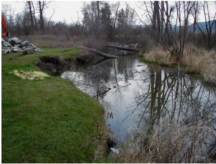
Figure 1: Eroding vertical bank on Dayton Creek prior to reshaping.
