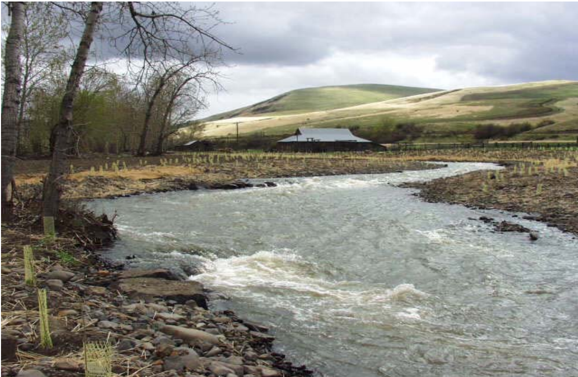
Photo 6. Upstream view (2002) of J-Hooks, reconstructed point bars and rooted stock plantings, implemented on the middle Houser property in 2001.
