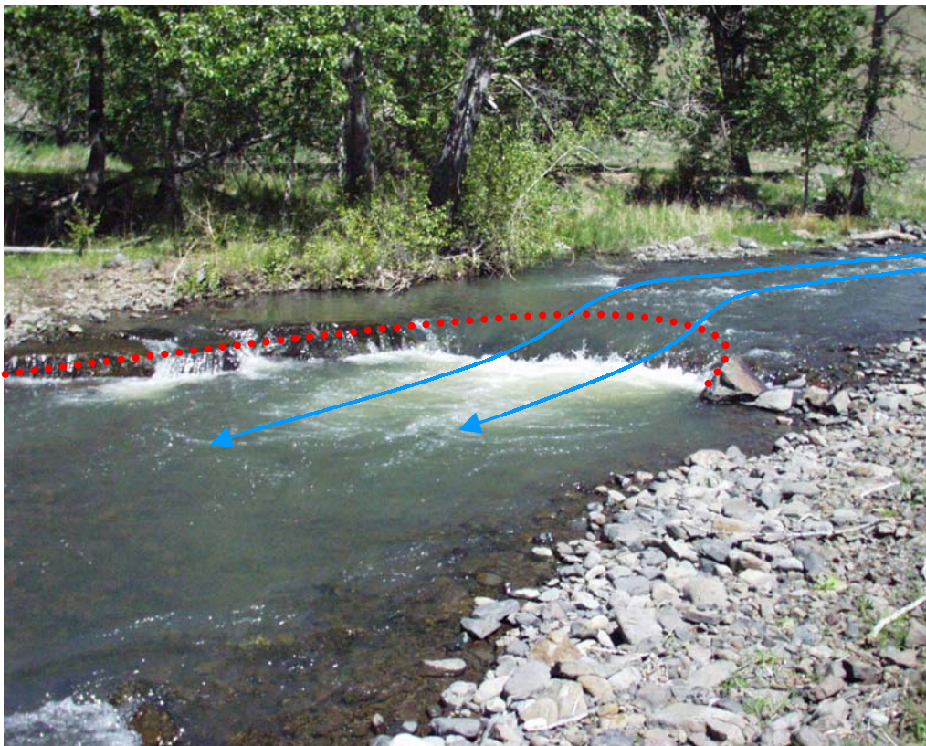
Upstream view of typical “J-Hook Vane” installed on the Brogoitti property (East Birch Creek), using Rosgen design principals and techniques.
