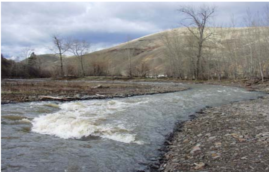
Photo 8. Downstream view (2002) of J-Hook structure and reconstructed point bar, implemented on the Brogoitti property in 2001.
