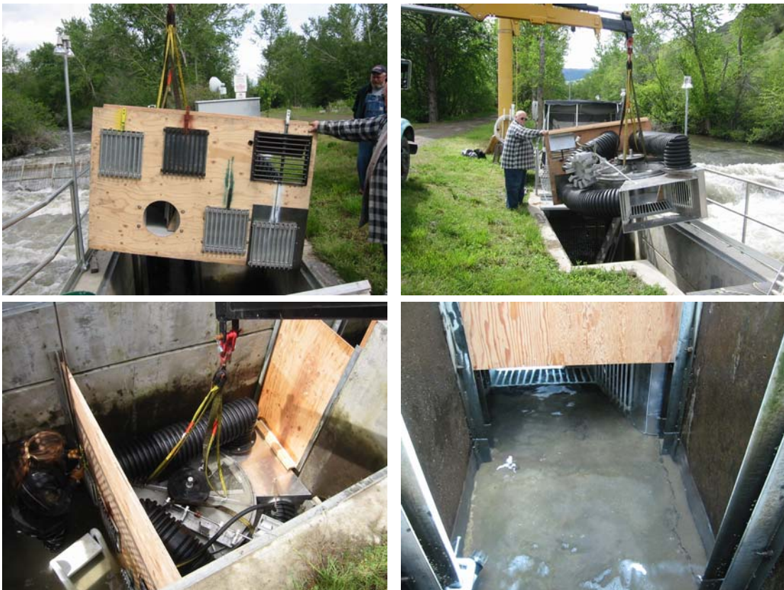
Figure 5. Fish passage device being installed in the fish ladder. From top left clockwise: upstream side of device showing attraction flow gates and exit (round hole), downstream side of device, entrance with no flow passing through device, top view of device installed (technician is on upstream side).
