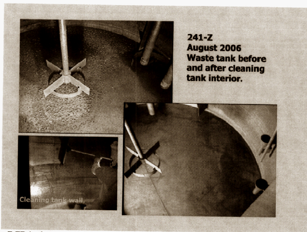
Figure 4 - RCRA closure activities: cleaning tank interior
