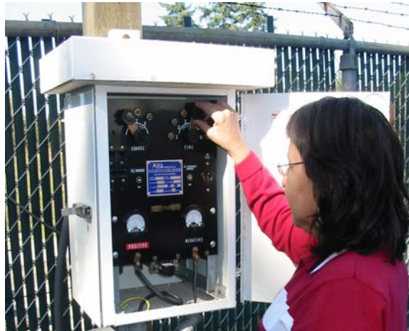
Figure 6 – Rectifier box for applying CP.
