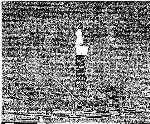
Figure 20: Solar power tower at the Solar Two power plant near Barstow, California. (U.S. Dept. of Energy, Sandia National Laboratory, <http://www.energylan.sandia.gov/sunlab/snapshot/powertower.htm>)
