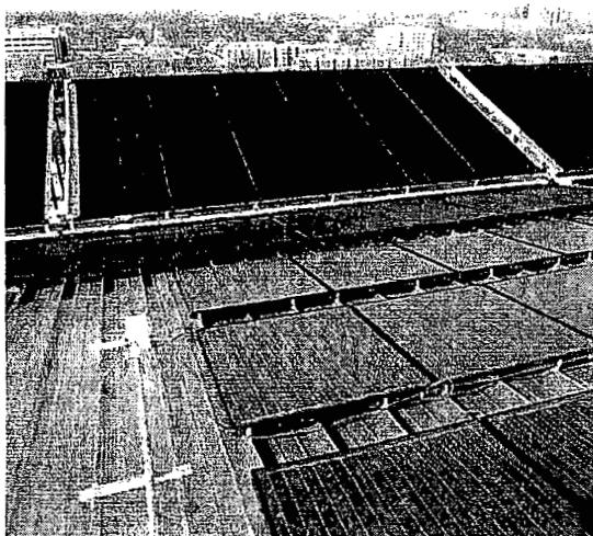
Figure 18: This swimming and diving facility uses photovoltaics (front) to produce electricity and a solar-thermal system (back) to heat pool water. The photovoltaic modules will provide 340kW of peak electrical power and will be the largest photovoltaic building installation in the world. Both systems will reduce demand on the local utility and result in significant annual energy and cost savings.(U.S. Dept. of Energy)
