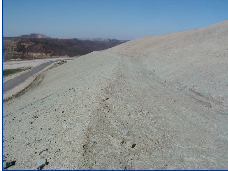
Figure 1.1. Example of a site prior to planting that exhibited a traditional grading practice (control).
