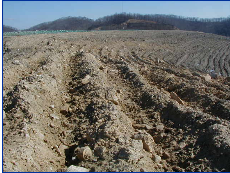
Figure 1.3. Example of a site prior to planting that has been ripped.
