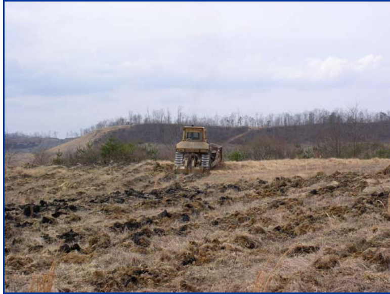
Figure 1.5. Example of a site that was reclaimed as pasture and is being ripped to alleviate the level of compaction in preparation for tree planting.
