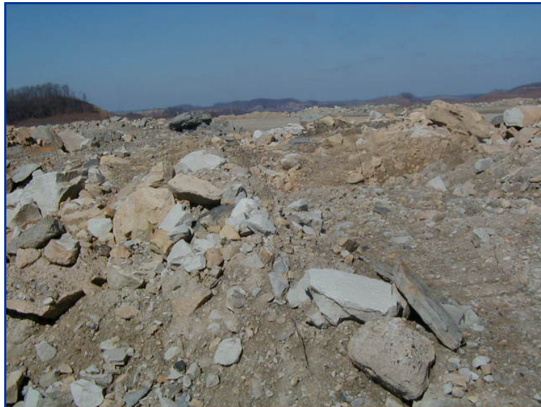
Figure 1.2. Example of a site prior to planting that exhibited the loose-dumped grading practice.
