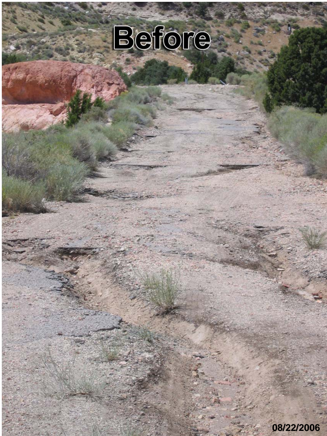
Figure C.1-2 CAU 551 Eroded Access Road Below B-Tunnel Area
