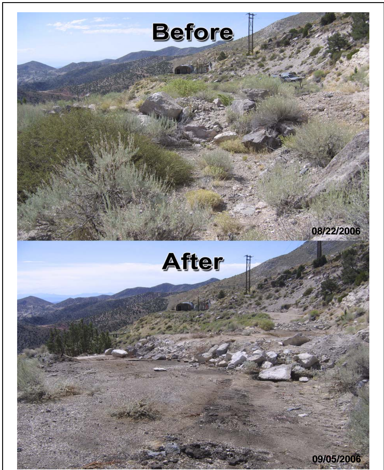
Figure C.1-5 CAU 551 Before and After Reconditioning of Upper Diversion Berm
