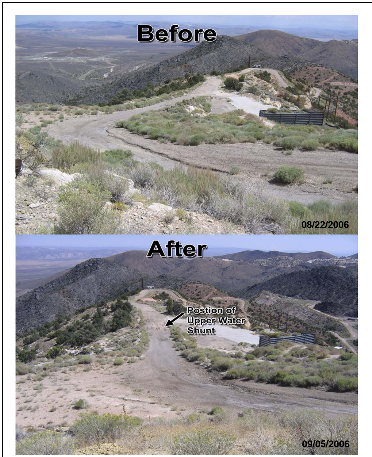
Figure C.1-7 CAU 551 Before and After Road Recontouring for Water Diversion
