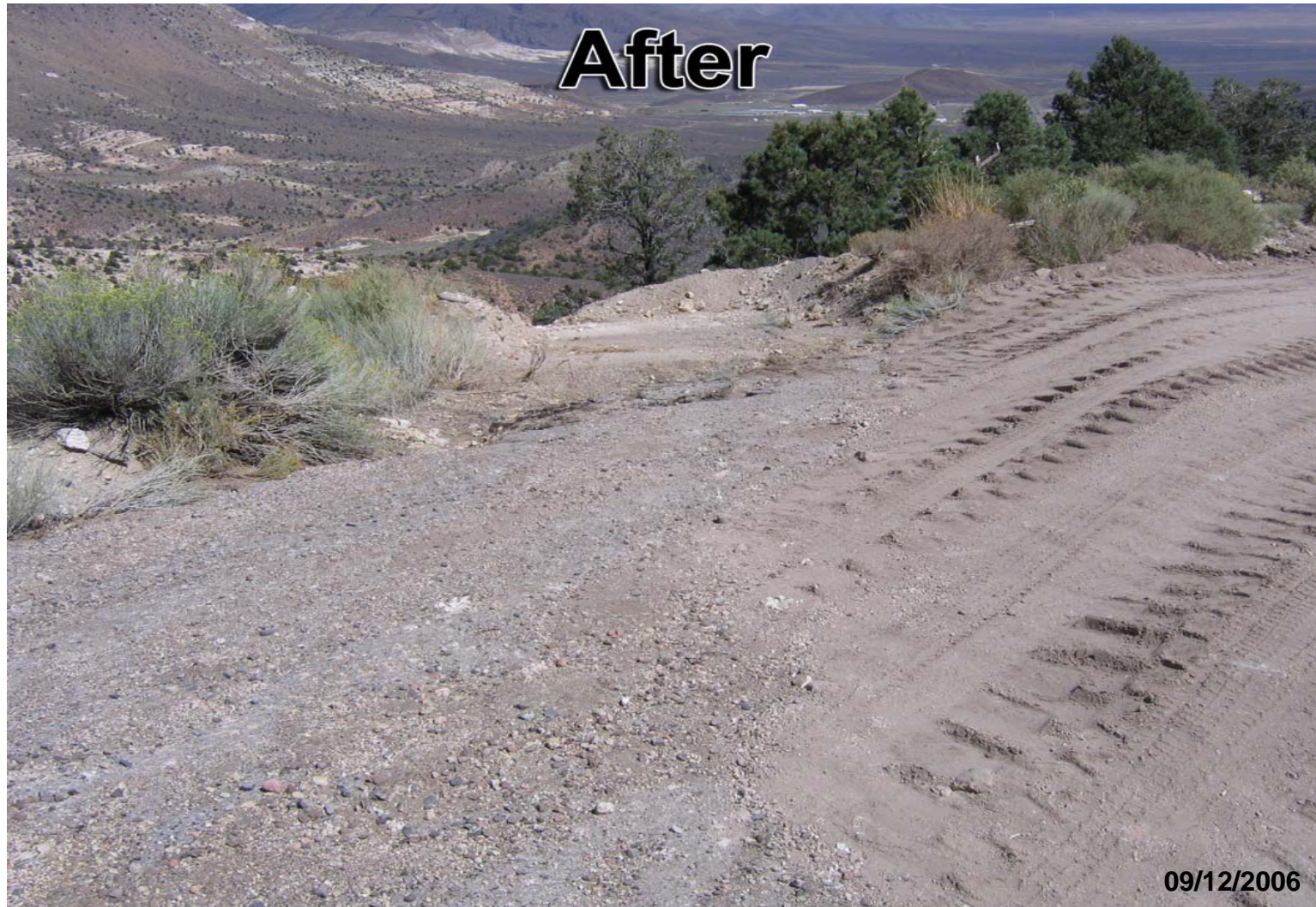
Figure C.1-8 Runoff Shunt on Access Road
