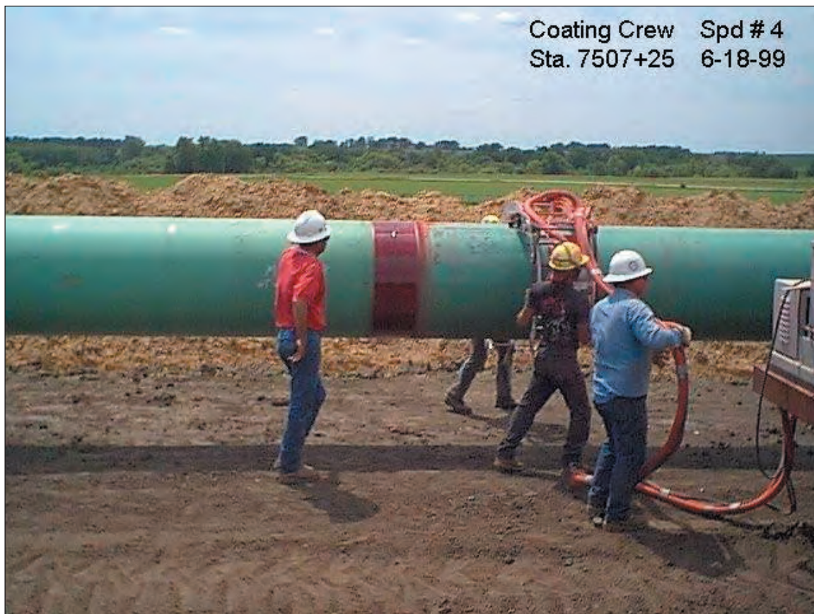
Figure C1.24. Coating using fusion bond epoxy
