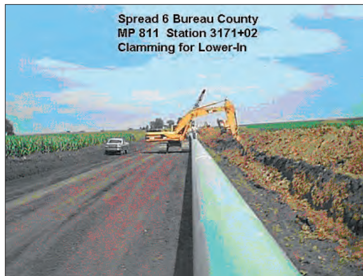
Figure 6.5. Backhoe reaches over pipe to clam out ditch
