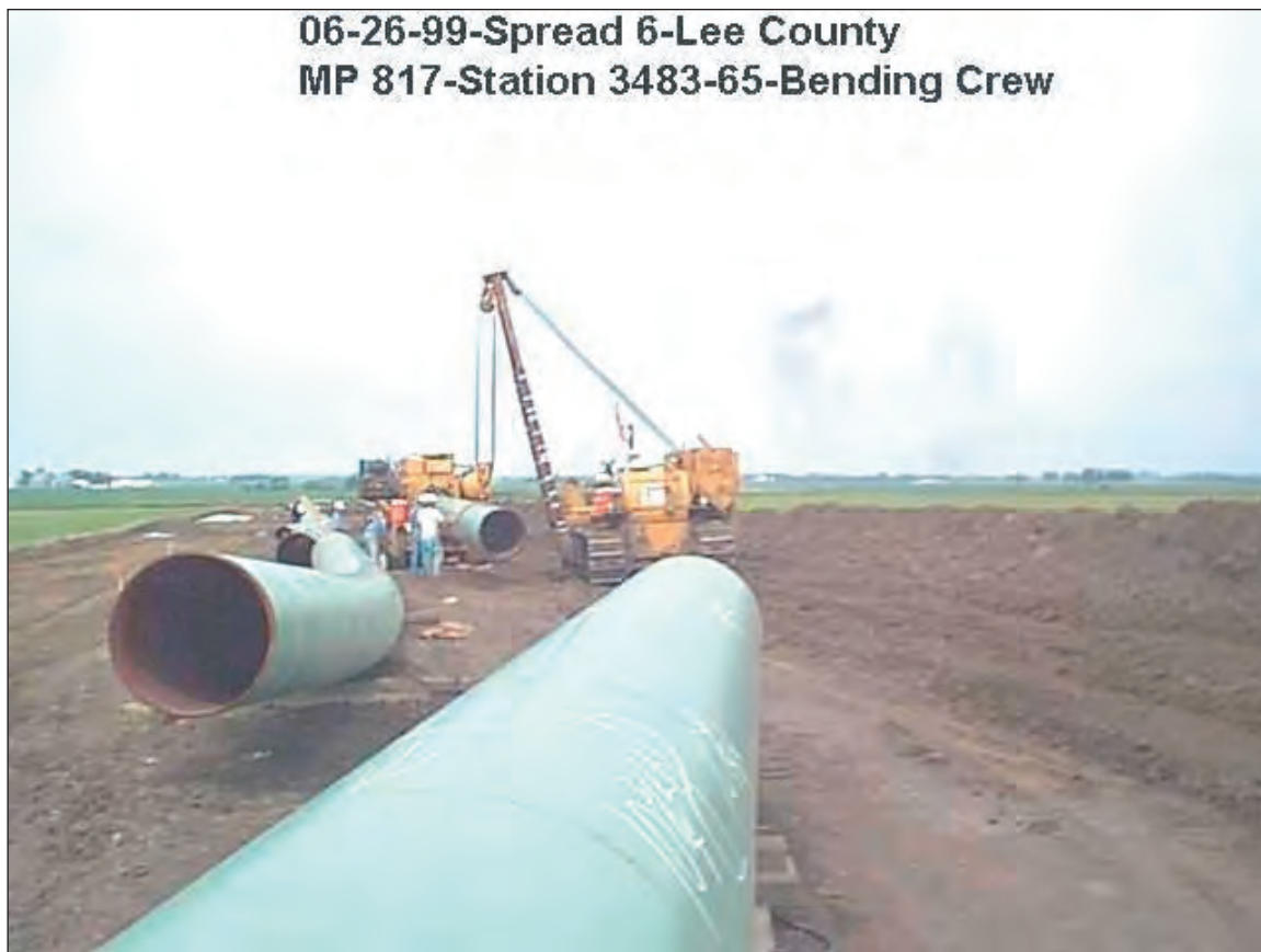
Figure C1.8. Pipe bent to accommodate direction change
