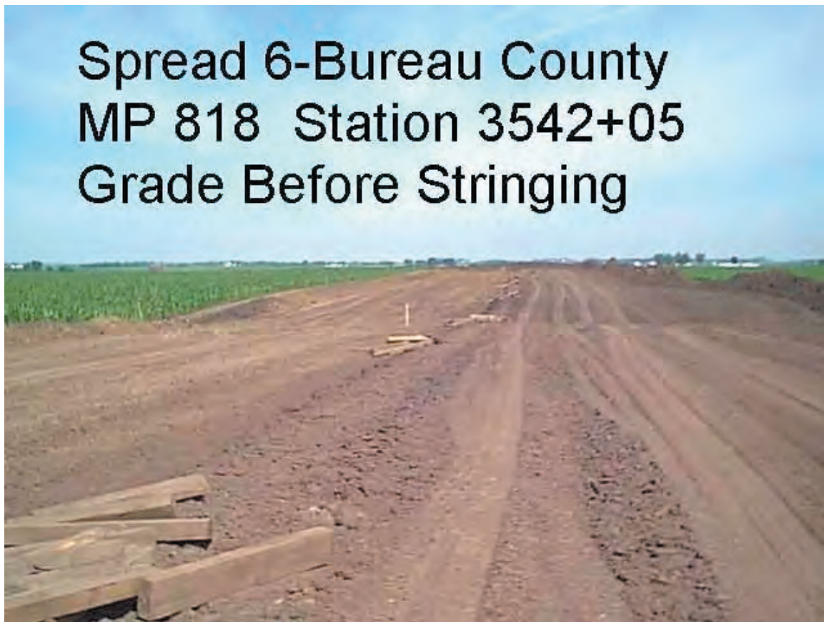
Figure C1.5. Completed grading. Note that the skids stringing, pipeline centerline stakes, and topsoil are stockpiled at the edge of the right-of-way
