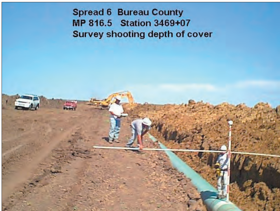
Figure C1.29. Surveying weld location and cover
