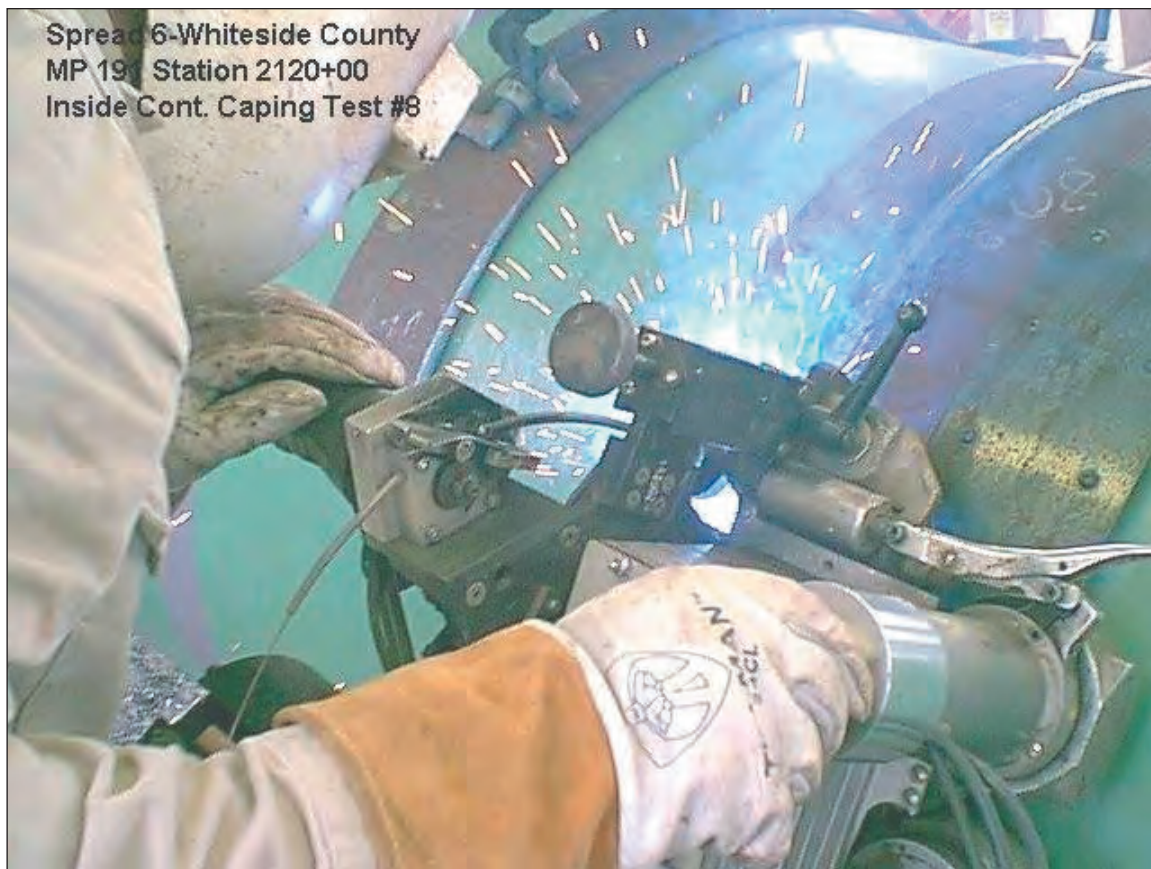
Figure C1.23. Mechanized welding, large-diameter high-pressure pipeline
