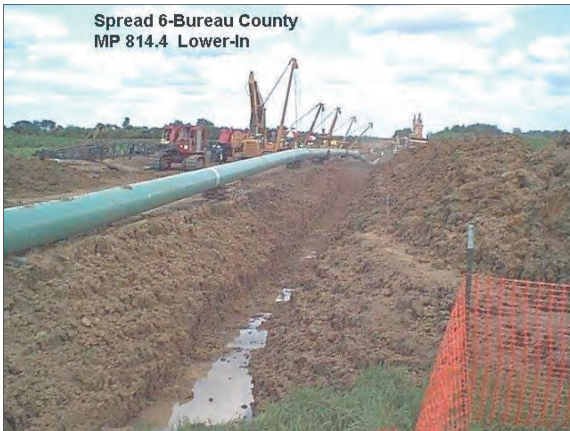
Figure C1.27. Lower-in tractors in various boom positions
