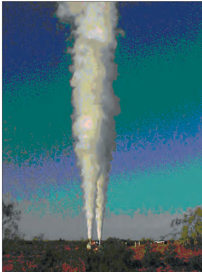
Figure 7.1. CO 2 venting from mainline block valve site
