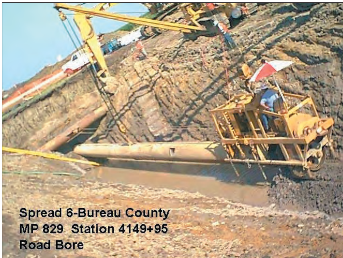
Figure C1.10. Road boring operation
