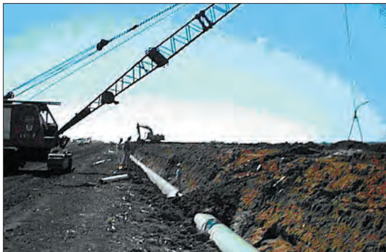
Figure 6.6. Crane plugs pipe during backfill operations
