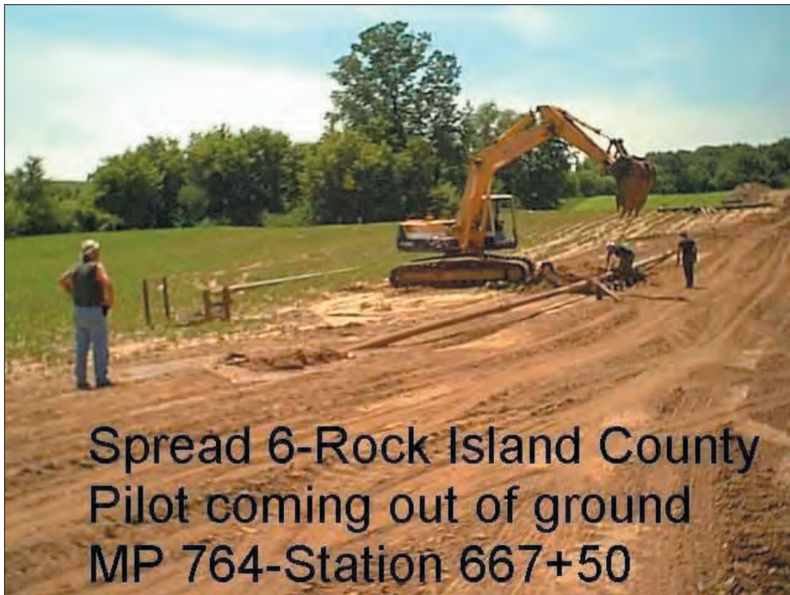
Figure C1.12. Horizontal directional drilling pilot coming out
