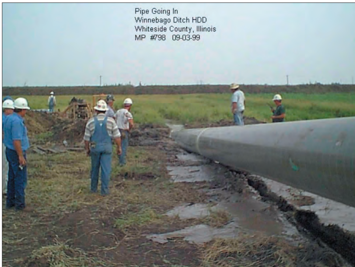
Figure C1.16. Pipe going in under levee canal
