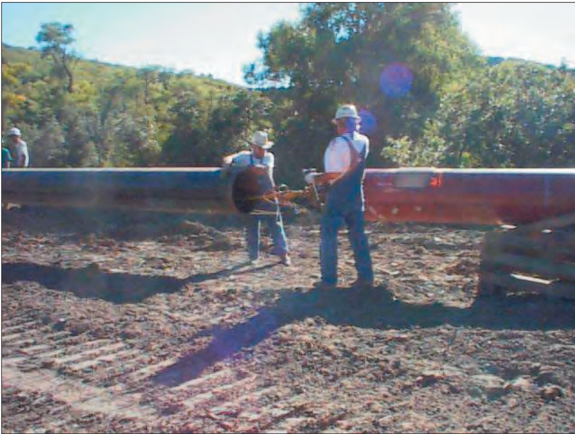
Figure C1.21. Pipe joint being stabbed over internal lineup
