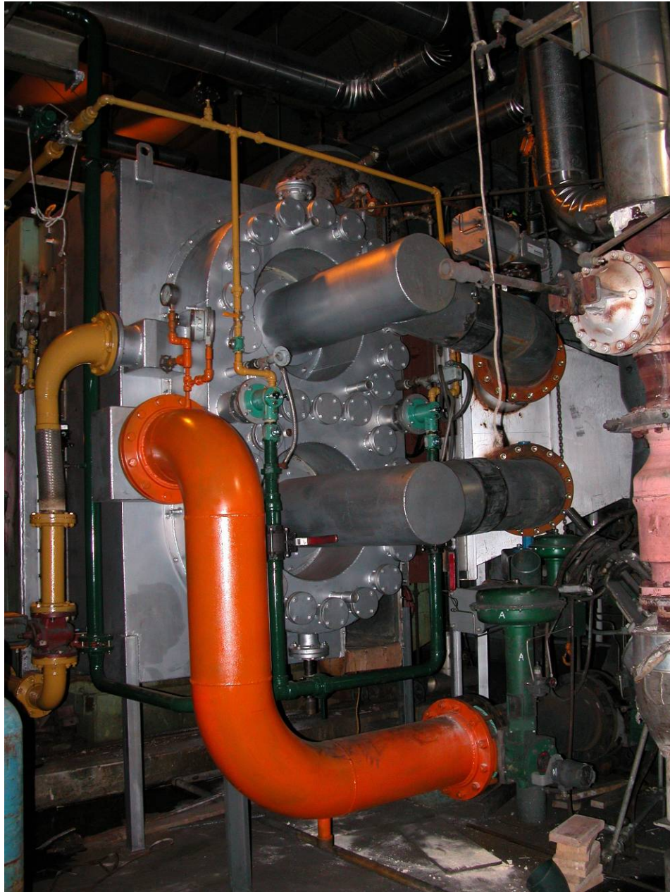
Figure 14. FIR BURNER INSTALLATION AT COKE-OVEN GAS BOILER SITE
