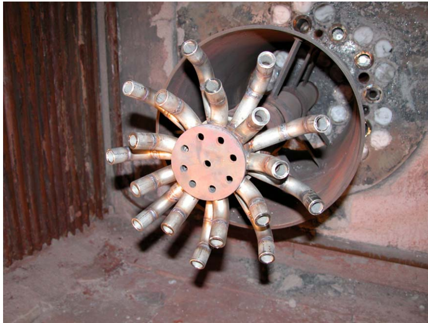
Figure 8. MODIFIED SECONDARY AIR TIP
