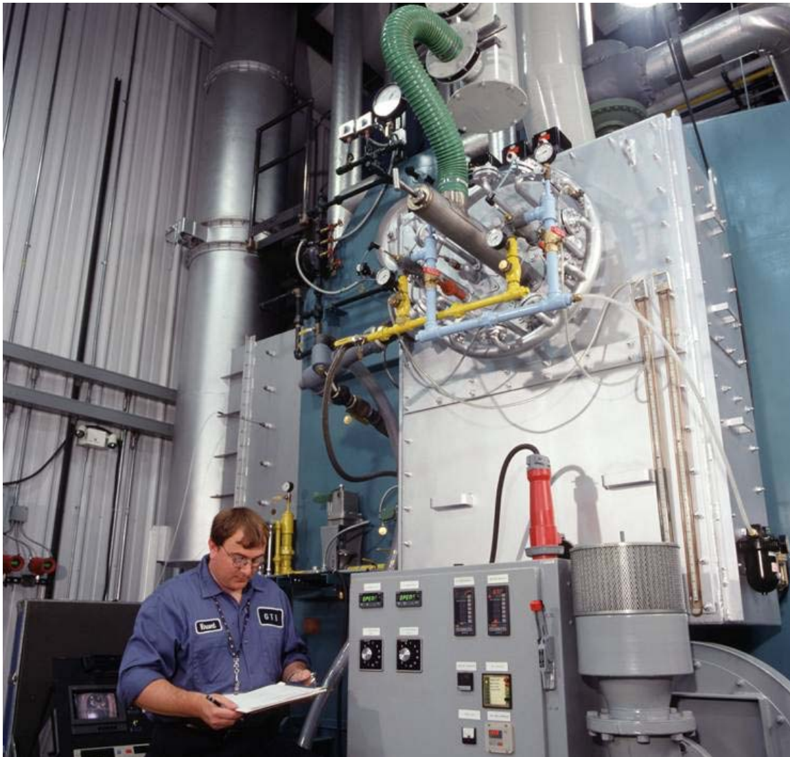
Figure 6. SINGLE BURNER PROTOTYPE ARRANGEMENT
