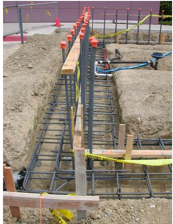
Image 9c: Rebar for CMU wall footing.
