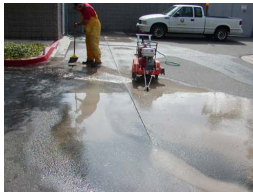
Image 5c: Saw cut for asphalt demolition.
