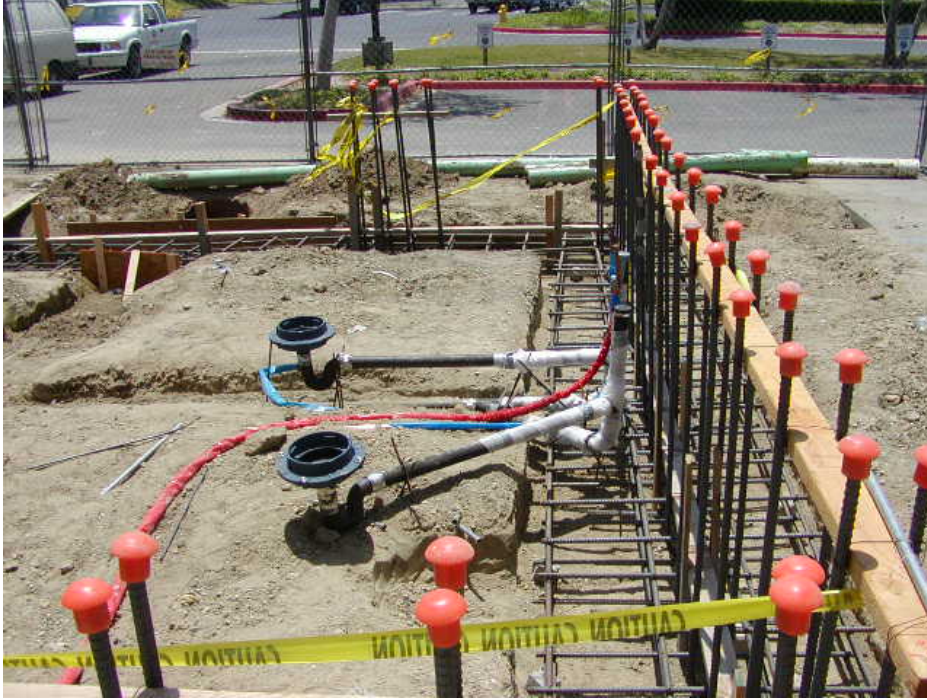
Image 9a: Drains that will be integrated into concrete slab, and rebar for CMU footing.
