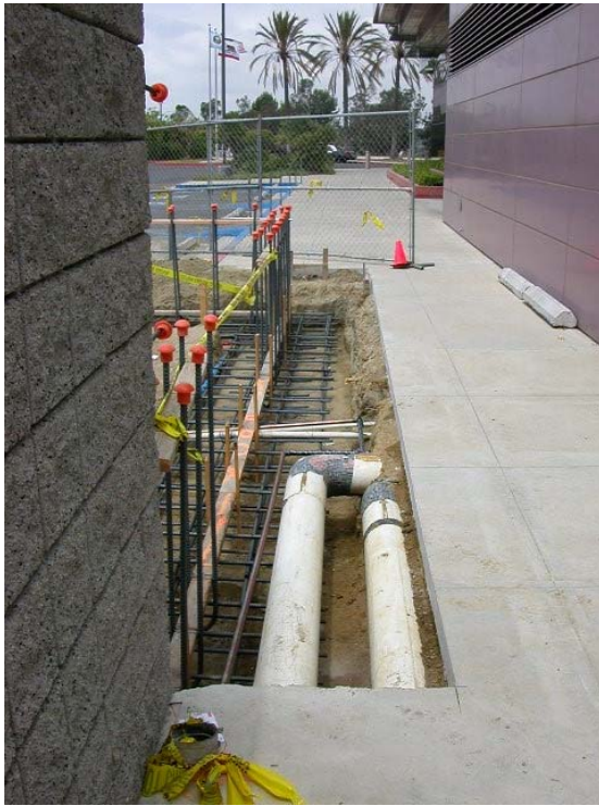
Image 9b: Trenching and support for CMU footing; existing chiller lines.
