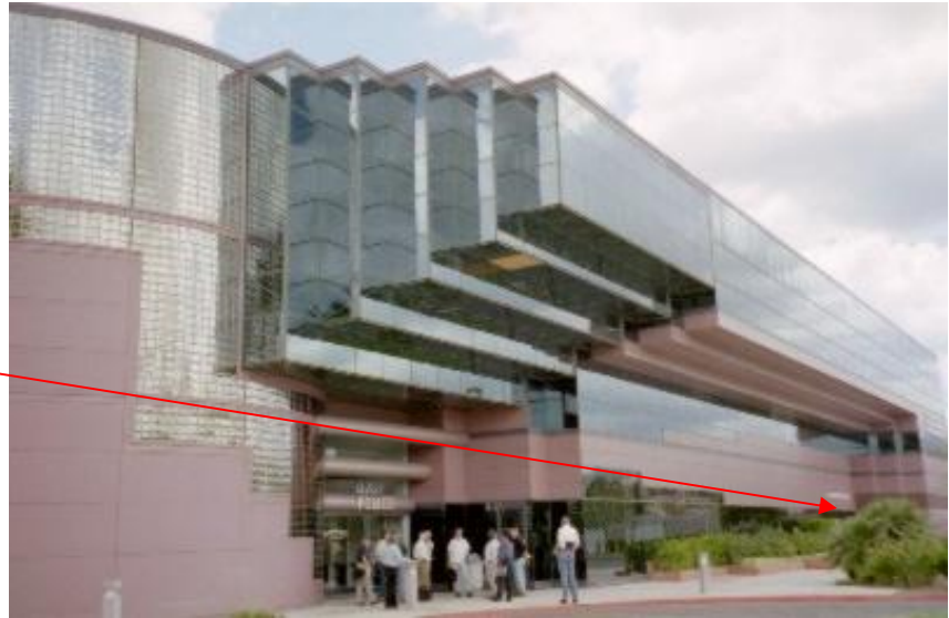
Image 1: Anaheim Police Department East Substation, 8201 E. Santa Ana Canyon Road in 2000. The facility is currently used for a Police Department on floors 1-3, with the Community Center on the ground floor at the East side of the facility.
