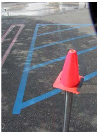
Image 5b: Saw cut for removal of parking space.
