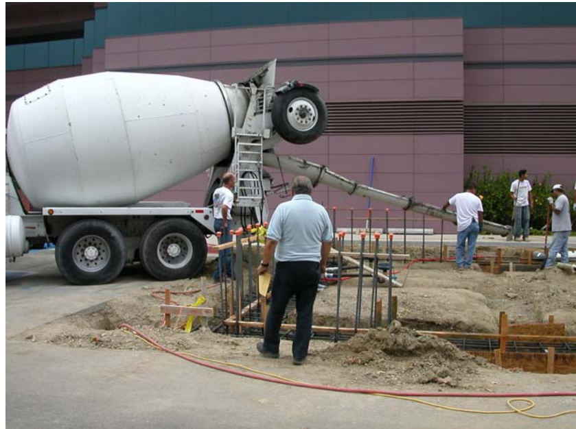
Image 13: Pouring concrete for CMU wall footing.
