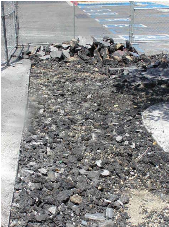
Image 8b: Demolition of asphalt.
