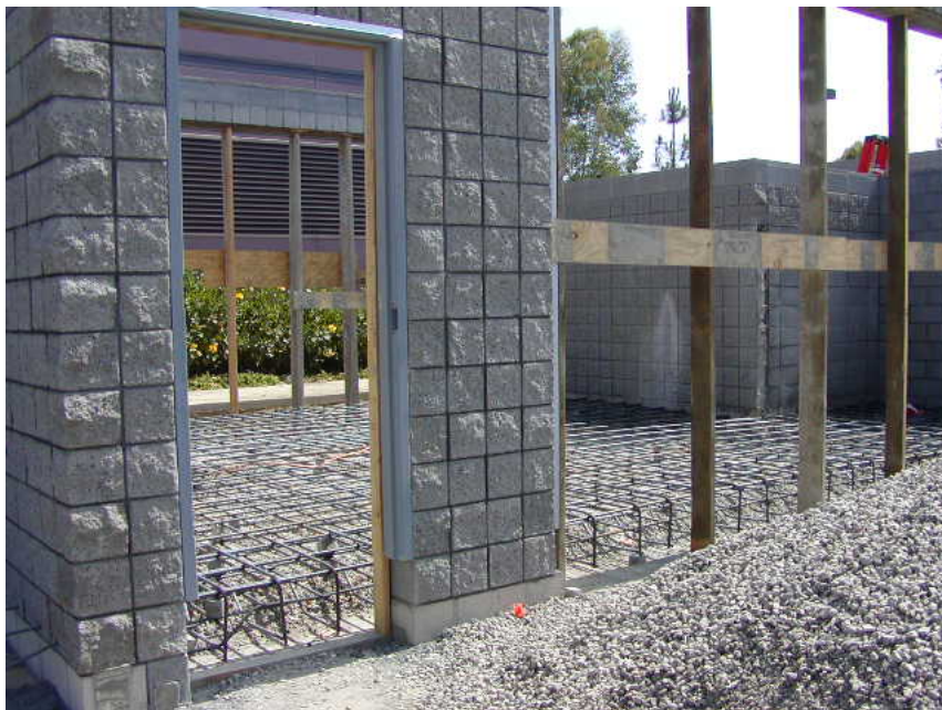
Image 14: Construction of CMU wall (June-July 2004).
