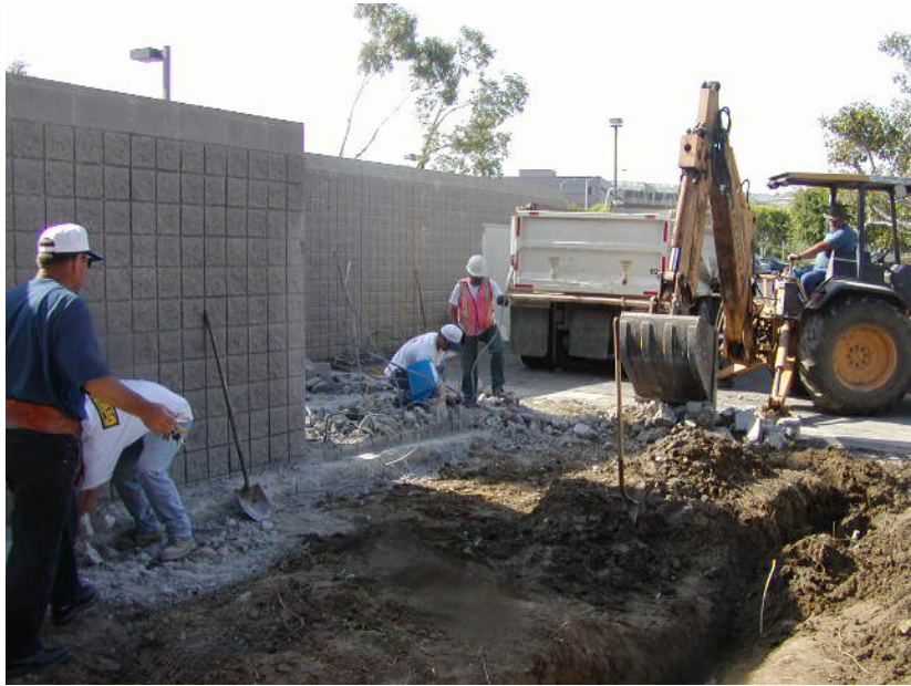
Image 8a: Demolition of original walkway and removal of tree.
