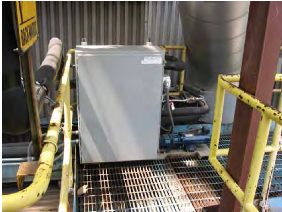
Photo 2-B. Metering Pump and Flowmeter Enclosure with 20" Flue Gas Extraction Tie-In in Background
