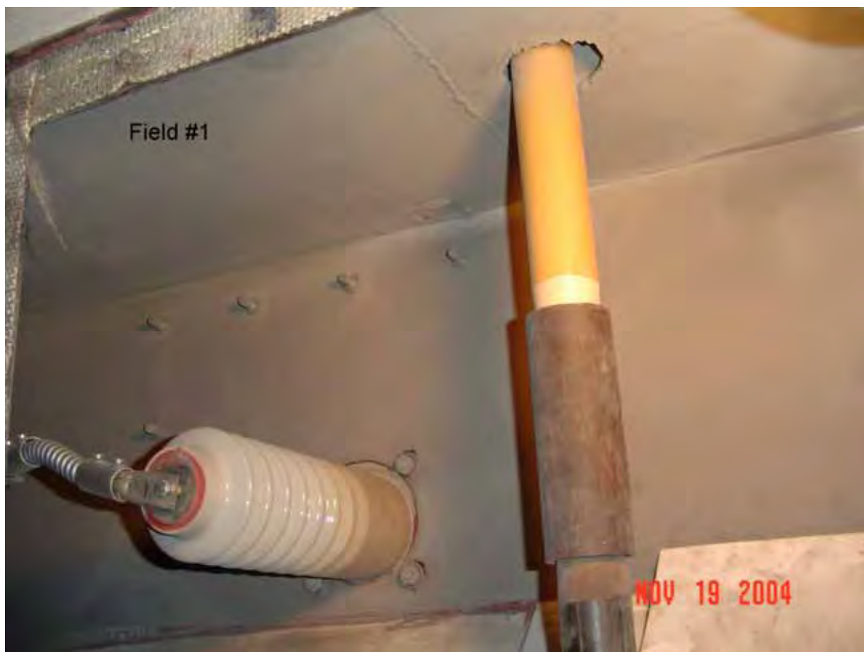
Figure 49. High-Voltage Compartment with Rapper Rod Insulator in Foreground, Wall Bushing and Teflon Barrier in Background
