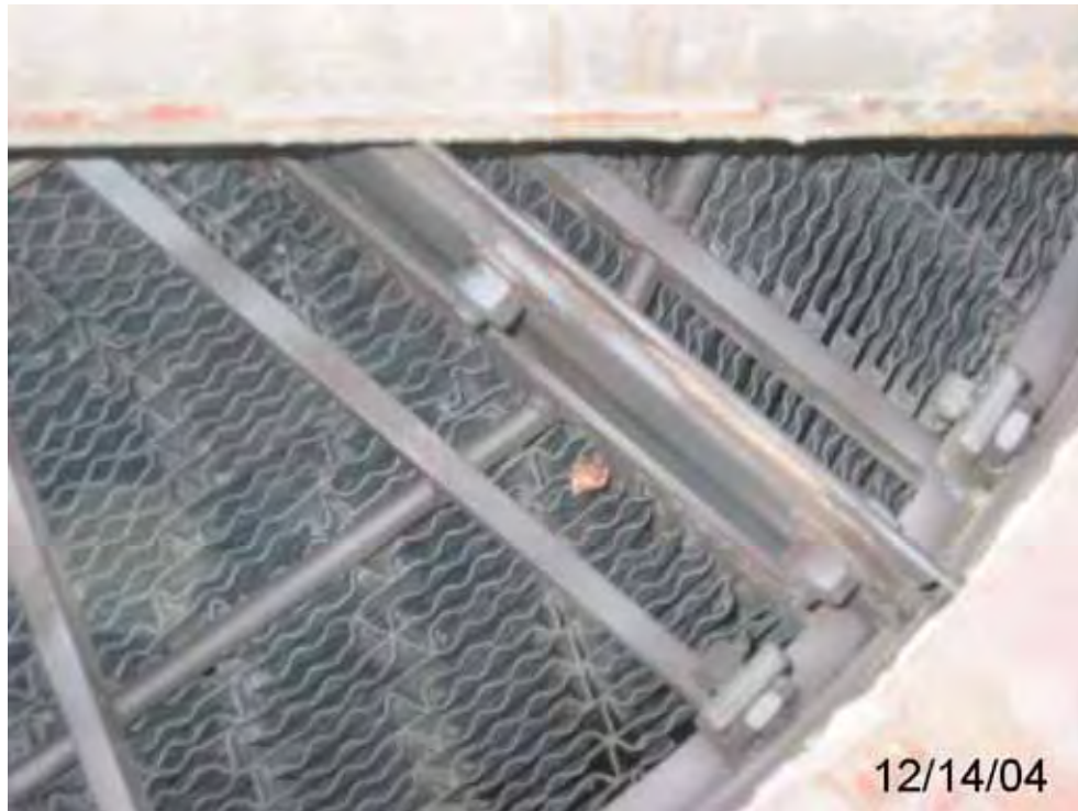
Figure 41. Cold End Basket After Soot Blowing
