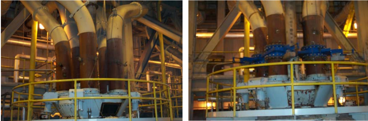
Figure 43 – Coal Balancing Valve Installation
