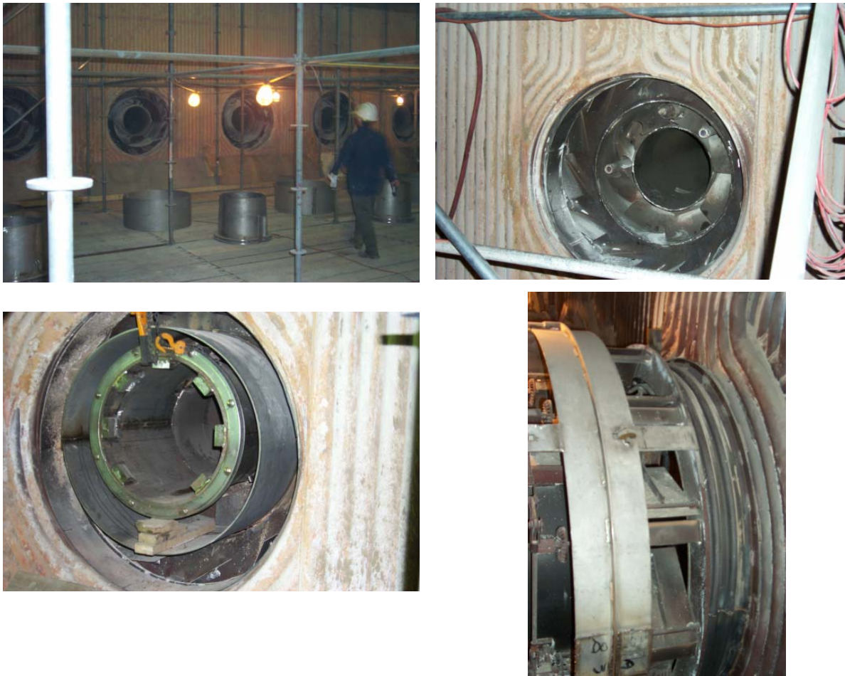
Figure 42 – Burner Modifications
