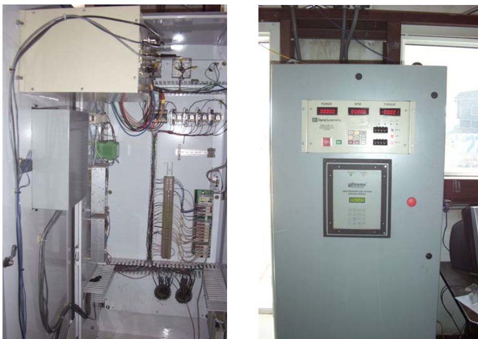
Figure 1. The data acquisition cabinet from inside (left) and outside (right).
