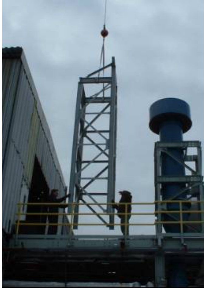
Figure 73. The cyclone and inlet pipe support installed on the burner deck
