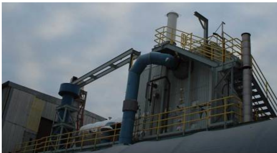
Figure 72. Cyclone support tower set on the CBTF burner deck
