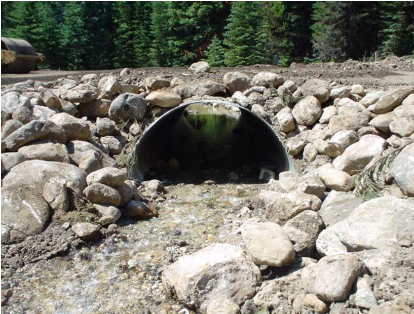
Figure 1. Inlet of the newly replaced culvert on Corral Creek.
