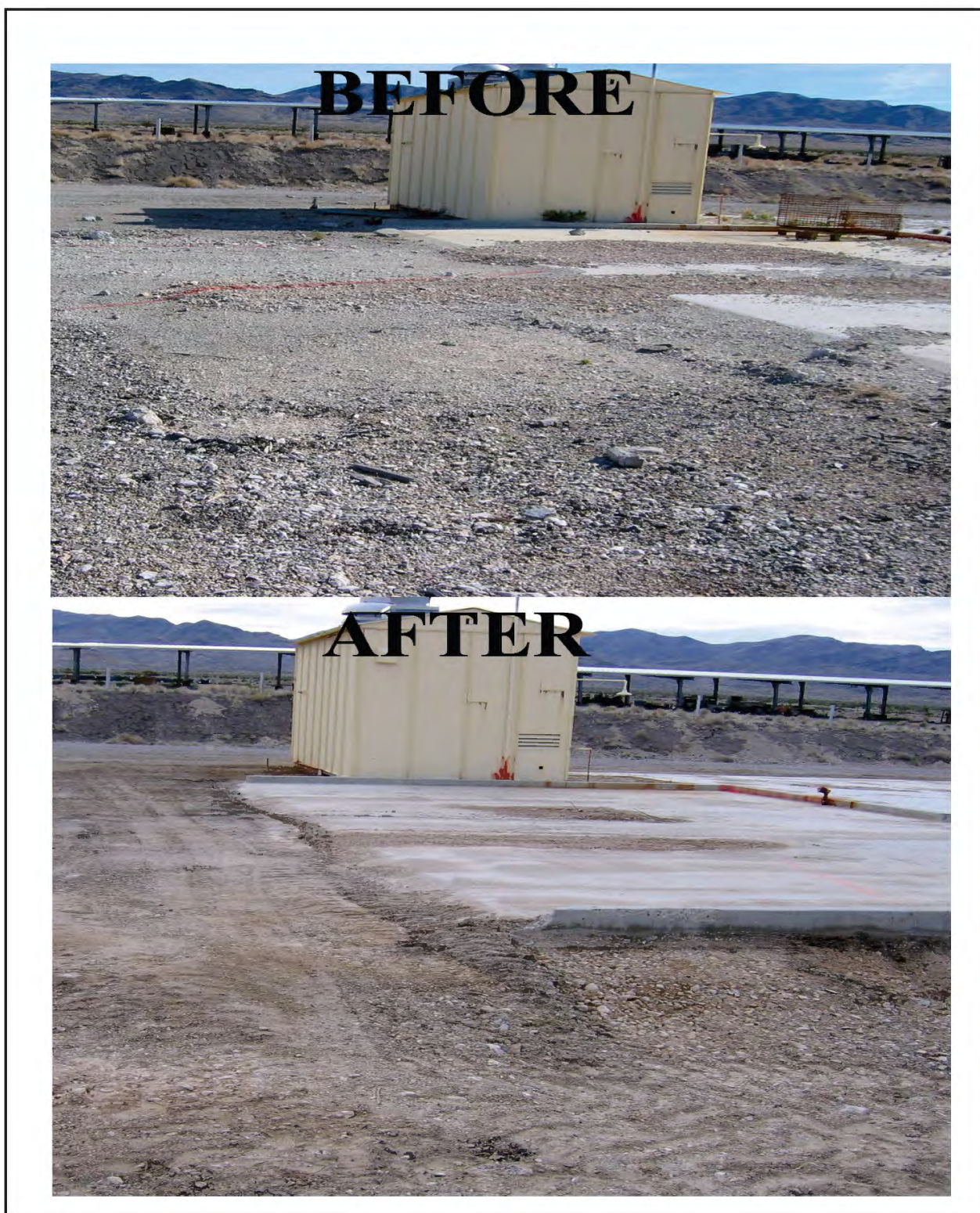
Figure D.1-11 CAS 23-20-01 North Side of Decontamination Pad (View looking east)
