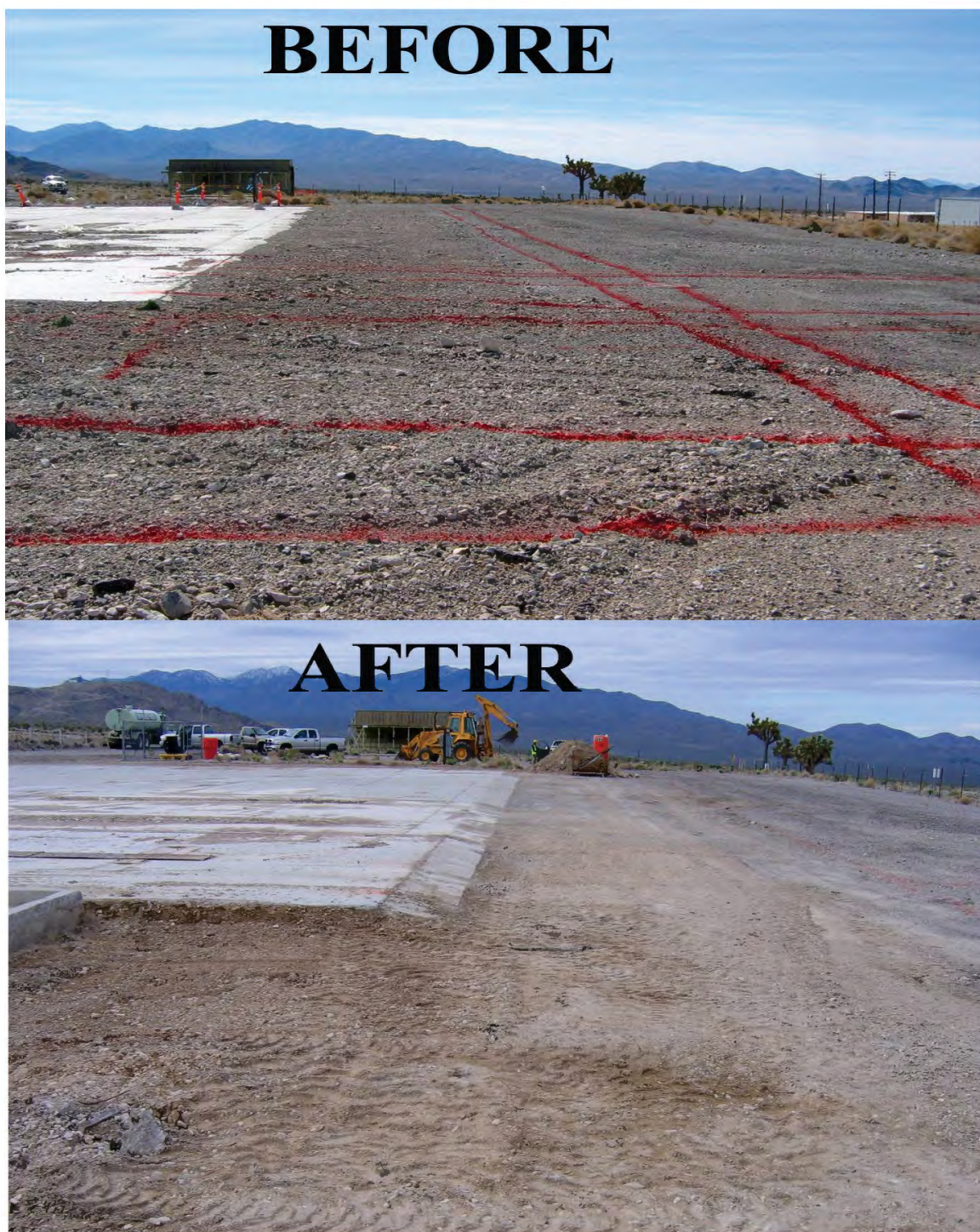
Figure D.1-10 CAS 23-20-01 Photos West Side of Large Concrete Pad (View looking south)
