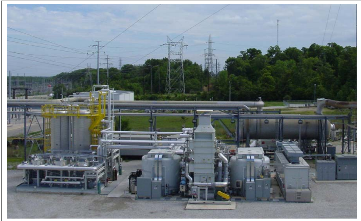
Figure 10-1. 2 MW Fuel Cell Power Plant With Syngas Processing Installed At The Wabash River Energy Ltd Gasification Plant in Terre Haute, Indiana
