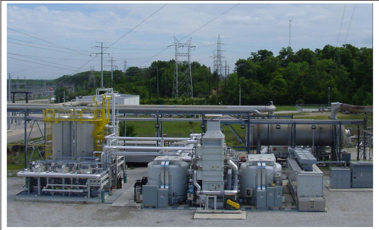
Figure 5-3. 2 MW Carbonate Fuel Cell Power Plant with Syngas Processing Skids Installed at Wabash
