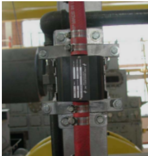
Figure 10-13 - Blow-by Flow Meter
