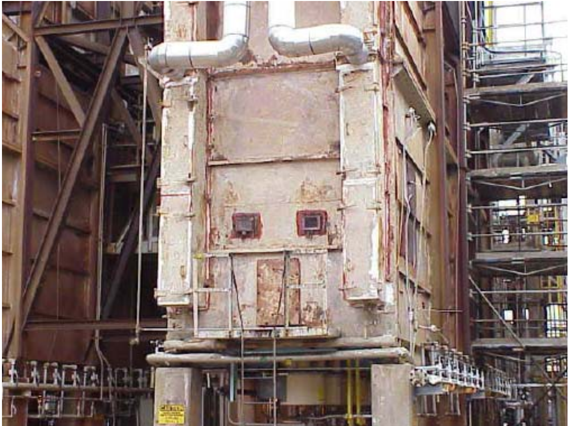
Figure 3-9. The Demonstration Heater for the Ultra Low Emission Burner
