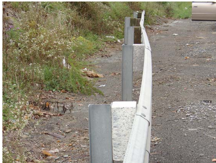
Figure 0-1 Guardrail offset blocks near Star city bridge, WV after 8 months of field installation
