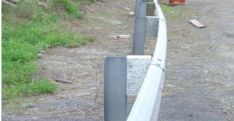
Figure 4-15 Guardrail system with polymer offset block
