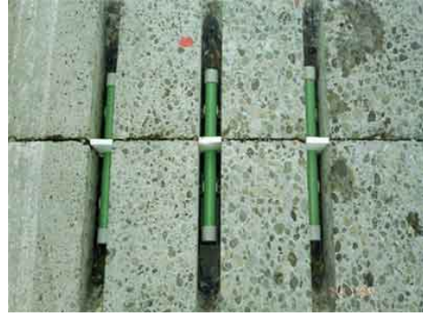
Figure 0-2 Dowel bars in concrete slabs
