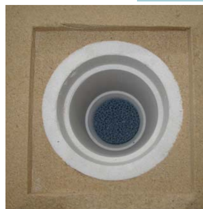
Fig. 10 Detail of the DPI sleeve without filling.
