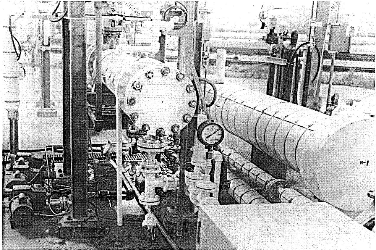
Figure 3: Titanium Heat Exchanger
