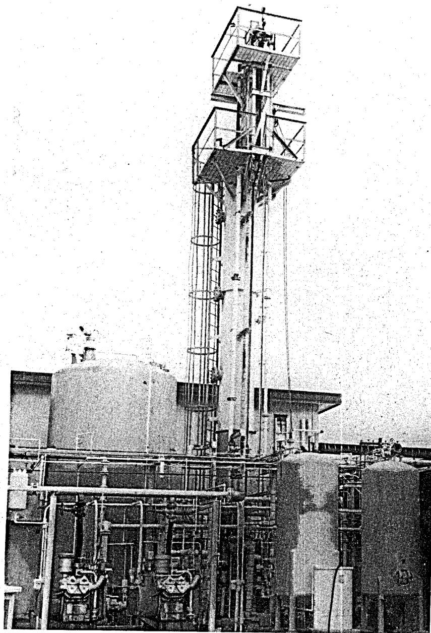
**Figure 2: Deaeration Tower and 10,000 Gallon Holding Tank.**
