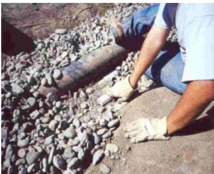
Image 6-2. Pressure tubes installed in LCRS trench
