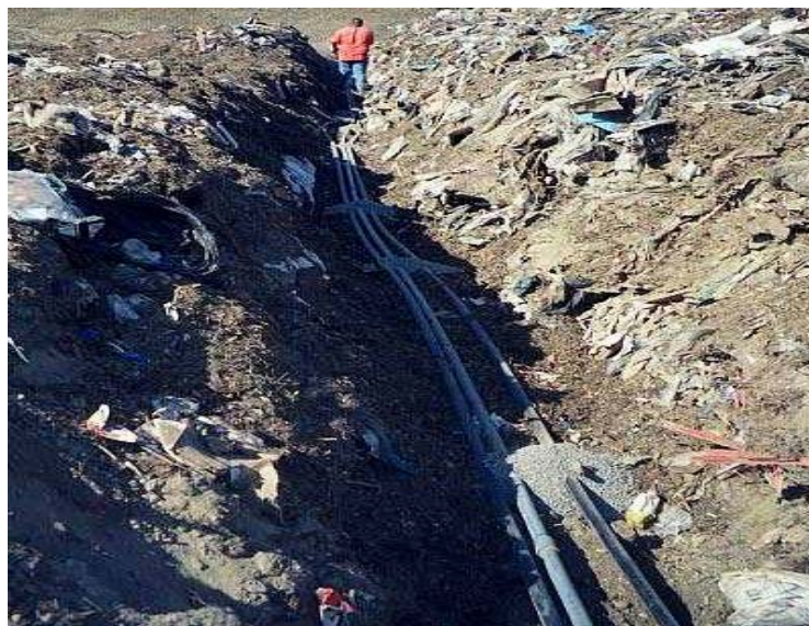
Image 5-2. Leachate injection laterals in trench
