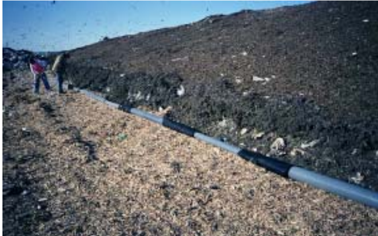
Image 3-2. Horizontal LFG collection line
