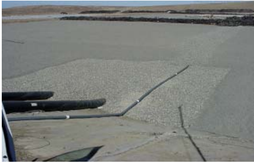
Image 3-5. Gravel drainage layer and leachate collection sump
