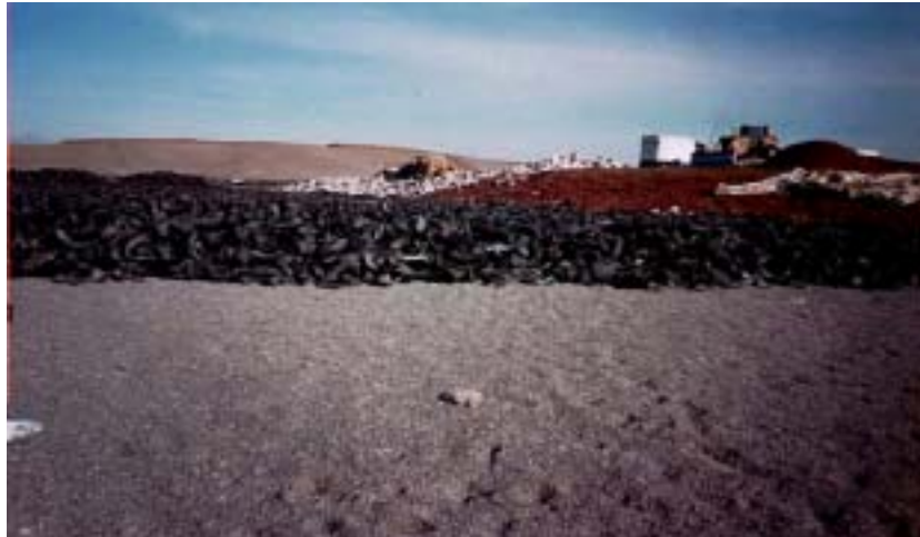
Image 6-1. Shredded tire operations layer
