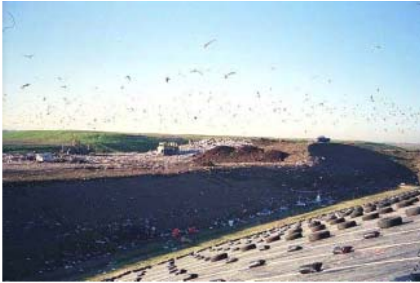
Image 4-1. Waste placement in the west-side cell
