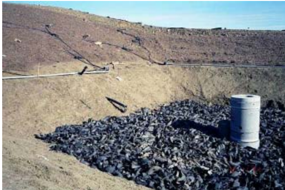
Image 5-4. Aerobic sump installed and ready for backfill
