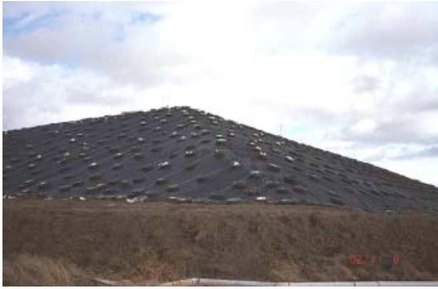
Image 4-4. West-side anaerobic cell surface liner.
