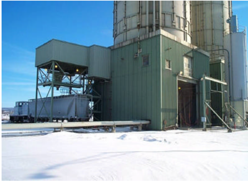
Figure 4.6. Montour Station Ash Handling System
