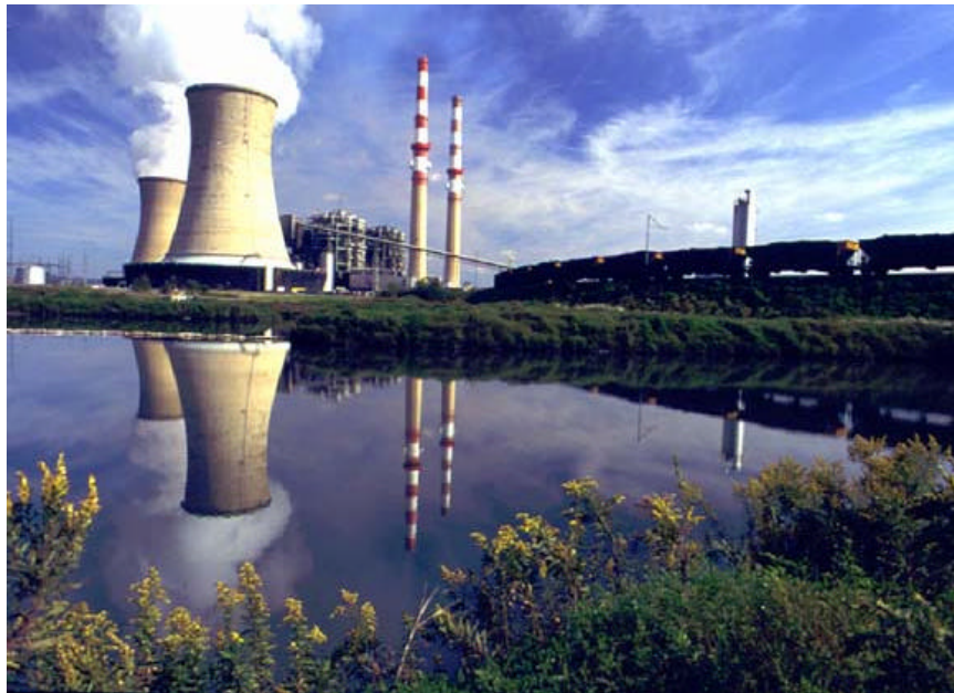
Figure 4.5. Montour Steam Electric Station
