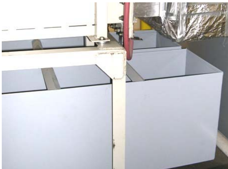
Fig. 3. Oil-Catching tanks installed under the high-voltage transformers.
