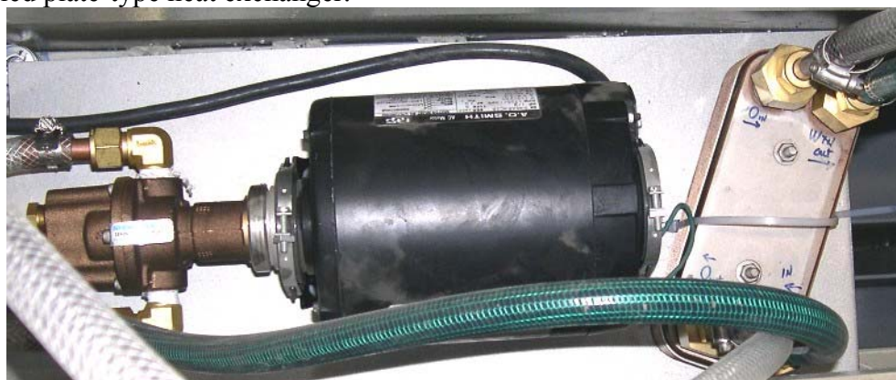
Fig. 4. Oil-cooling system elements installed between the high voltage transformers: the oil pump and plate-type heat exchanger.
