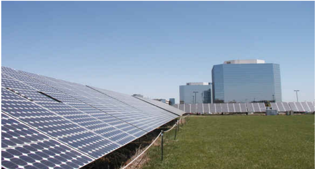
Southfield's 26kW Siemens Solar, which is located internal to Distribution Circuit 9010 fed out of the Southfield substation.
