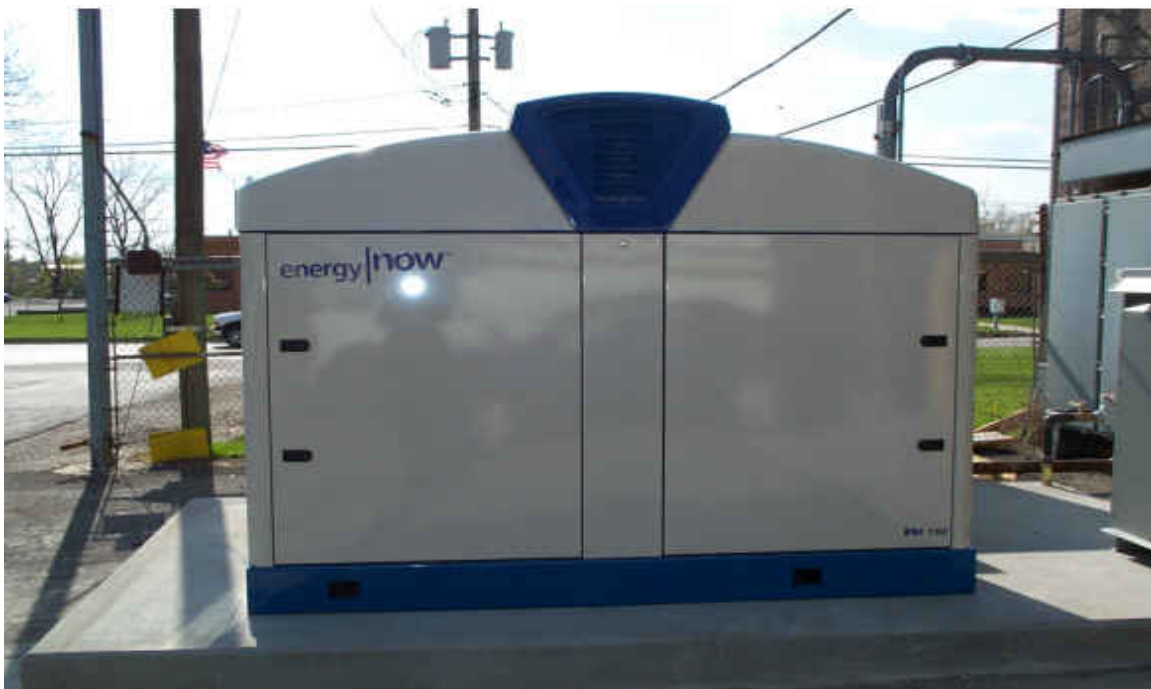
Farmington's 75kW ENI 75 natural gas internal combustion generator, which is located internal to DC 9016 and fed out of the Sunset substation.
