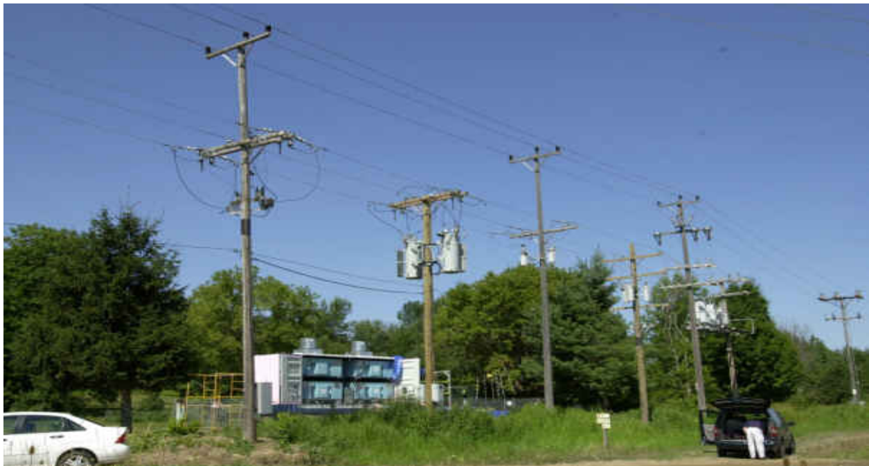
ZBB/SANDIA 200kW Flow Battery, which is located internal to the 4.8kV delta DC 2628 fed out of a pole, mounted at the substation STDF4 (Sub Transmission Pole Mounted Distribution Facility) in Lum, MI.
