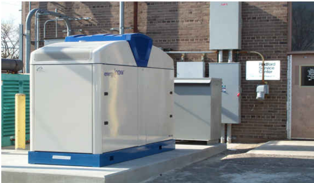
Redford Service Center's 150kW ENI 150 natural gas internal combustion generator, which is located internal to DC 561 and fed out of the Glendale substation.
