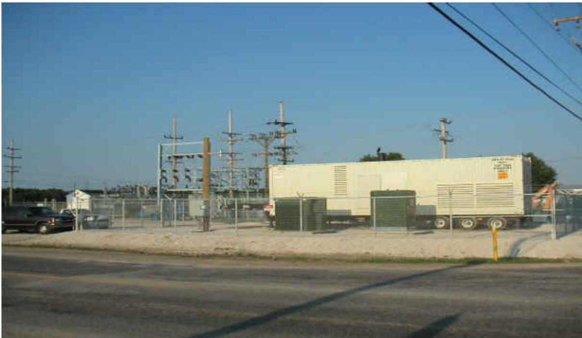
Adair substation has an ENI 1000, which is a 1MW natural gas Deutz generator. The generator is owned by Detroit Edison and feeds into the Adair 4.8 kV distribution circuit DC 322.
