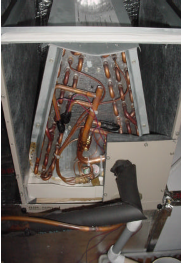
A-frame coil arrangement
