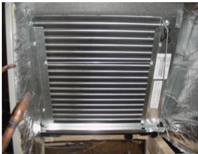
Slanted coil arrangement
