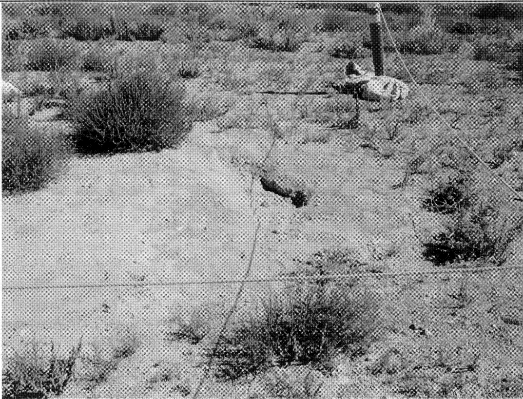
9. Subsidence area along east side of cover.
