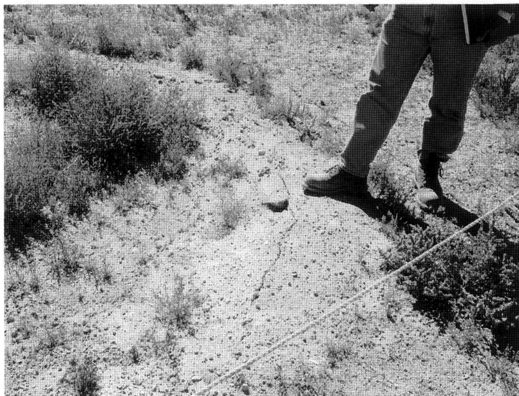
12. Subsidence area along southeast side of cover.
