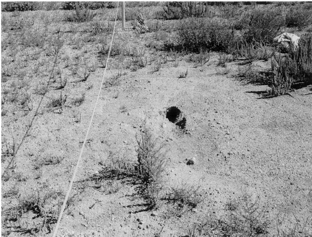
10. Subsidence area along east side of cover.
