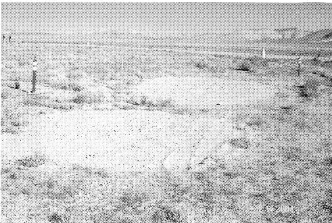
10. Two repaired areas along southeast side of cover.
