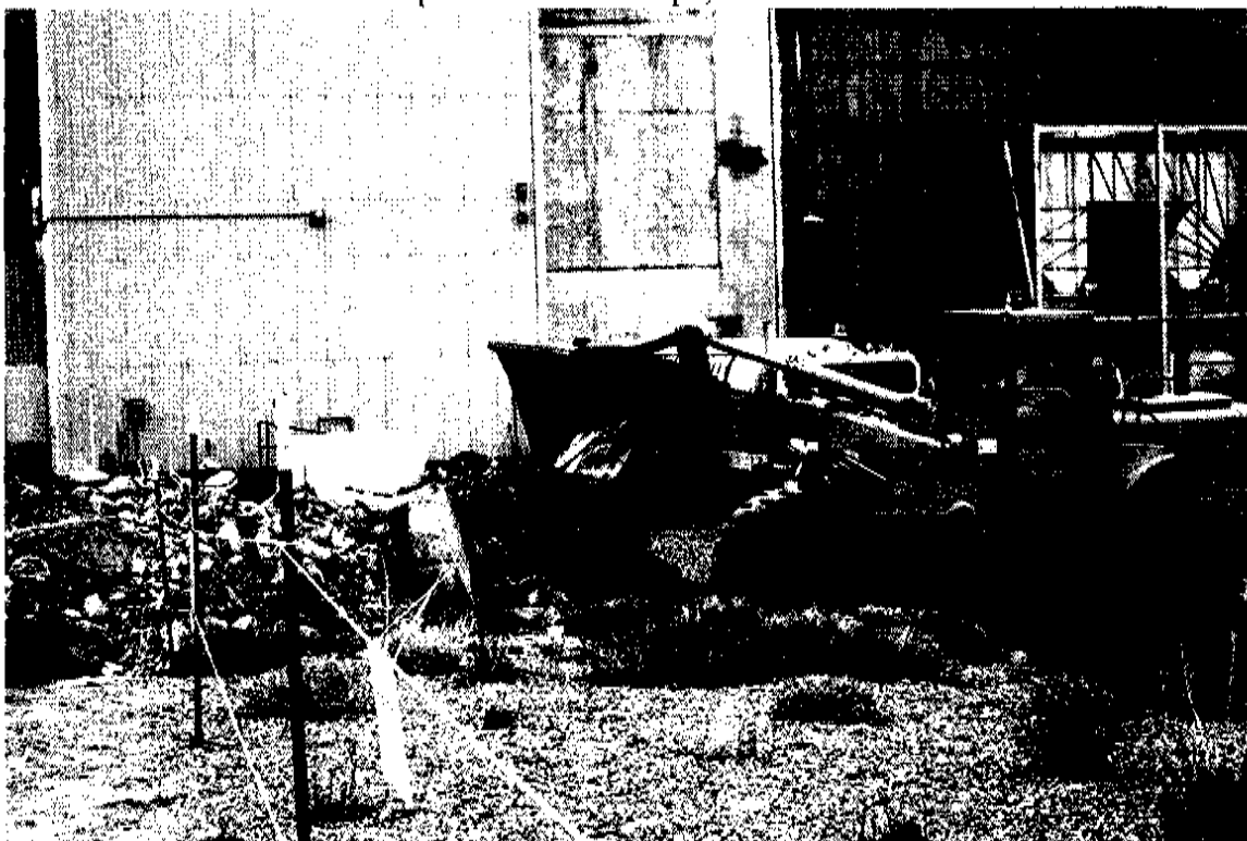
Photograph 3: CAS 25-07-06, Train Decontamination Area, Rubbilization of Concrete Pad, 03/04/2005
