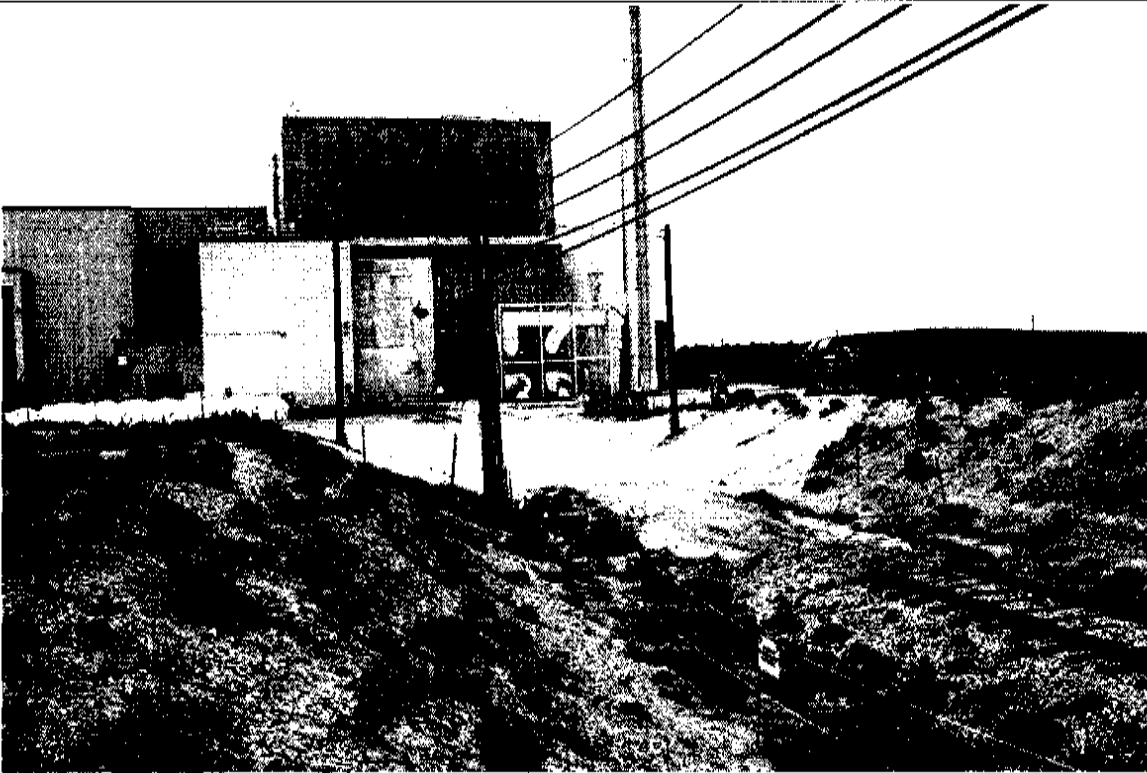
Photograph 10: CAS 25-07-06, Train Decontamination Area, Closure Activities Complete, Before Disposal of Low-Level Waste, 04/07/2005
