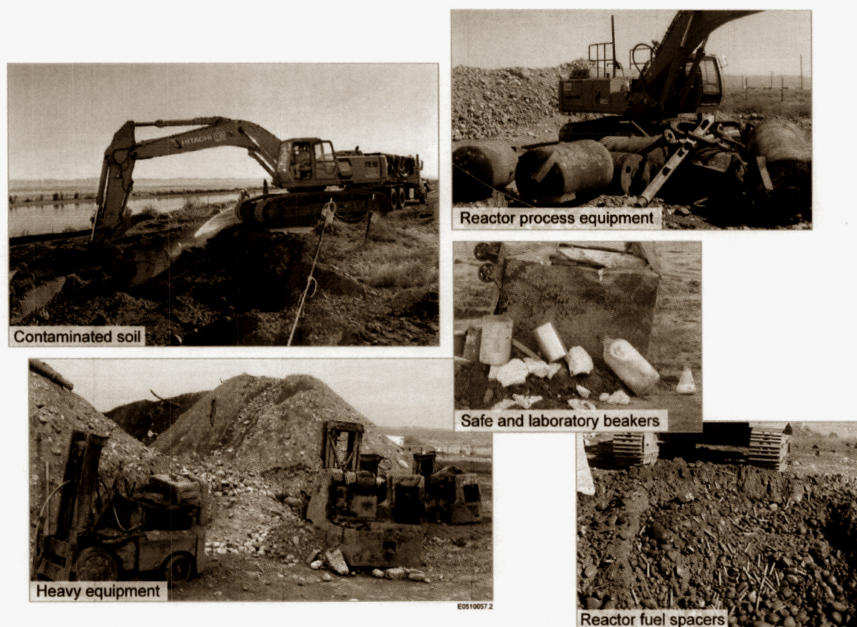
Fig. 3. Excavation of contaminated material from waste sites and burial grounds near the Columbia River
