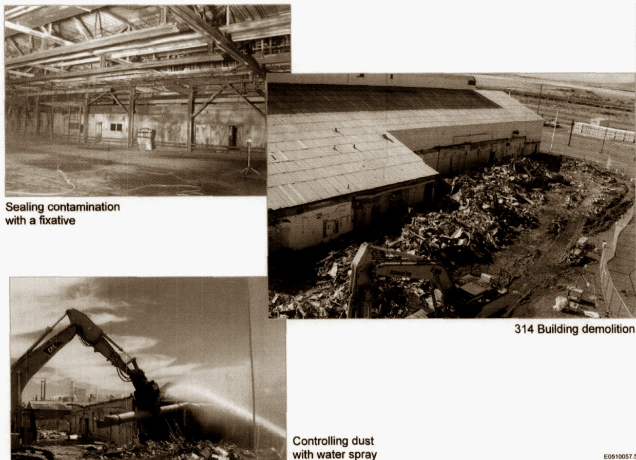
Fig. 2. Eliminating the spread of contamination during facility demolition
