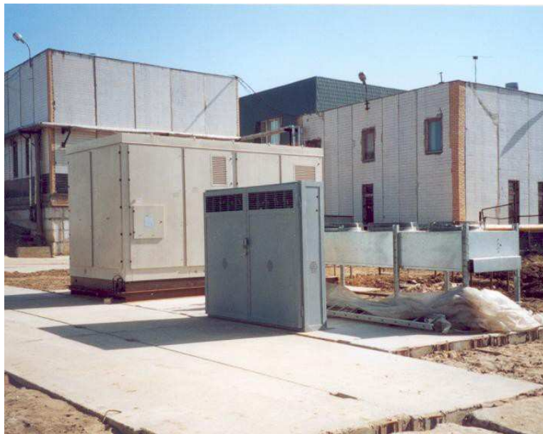
Figure 1 - Installation of PC25 at Orgenergogaz Facility near Moscow
