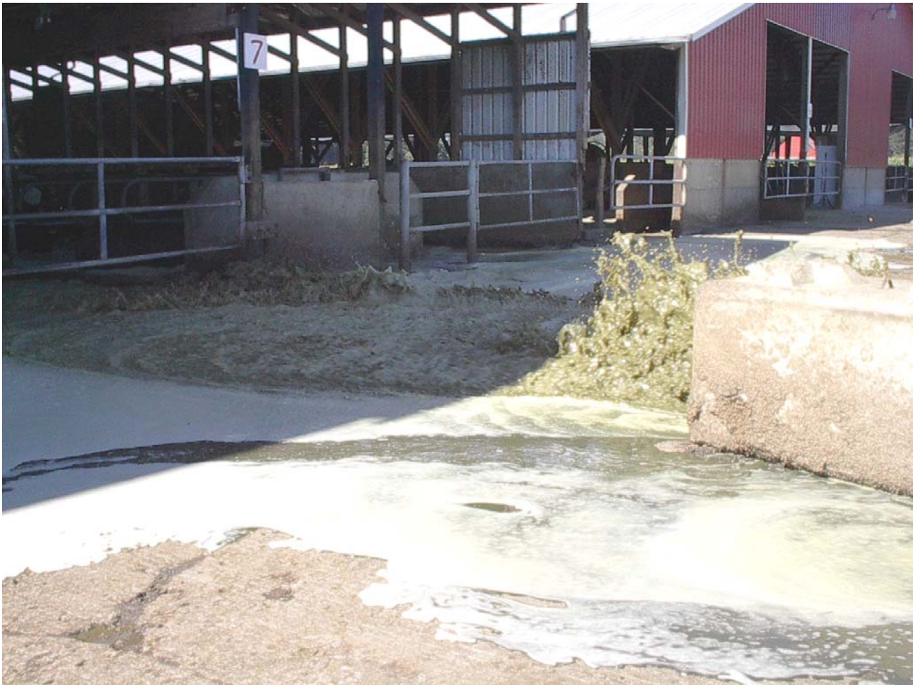
Figure 5. Flushed Manure Collection System
