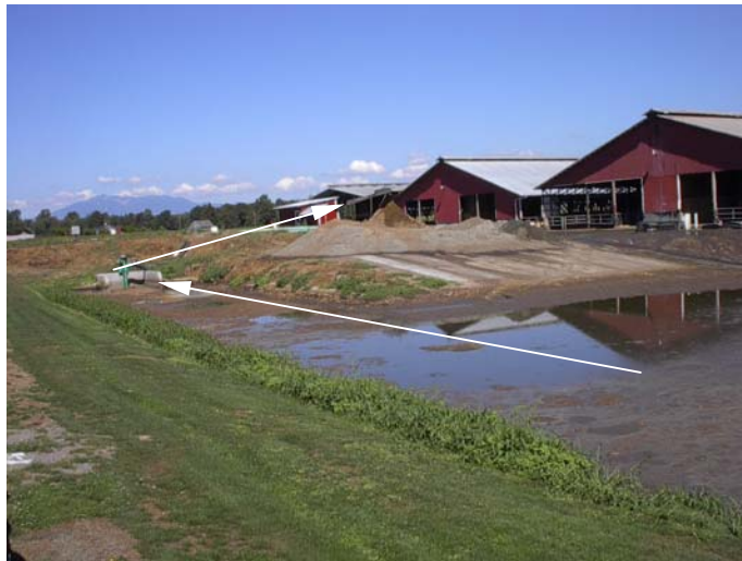
Settling basin liquid flows to pump and then to separator
