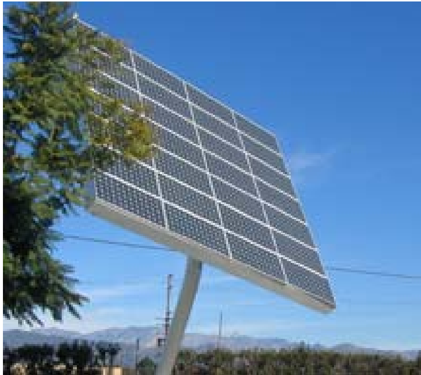
Figure 5-16. Pole Mounted Two Axis Tracking PV Array 4
