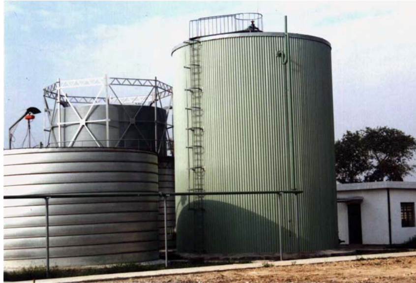
Figure 5-18. 500 m 3 Digester Treating Manure from a 10,000 Pig Farm in China. 7
