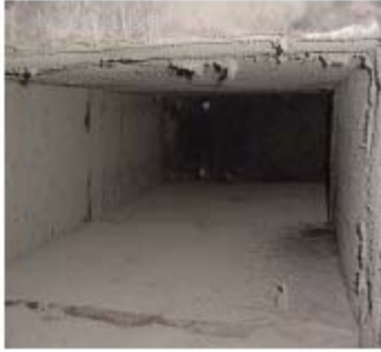
Figure 7: Dust in return duct after outside air intake
