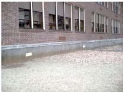
Figure 7: Unit ventilator outside air intakes at the Oregon Elementary School #1.
