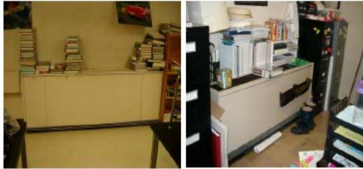
Figure 8: Unit ventilators at Minnesota school partially blocked by books.
