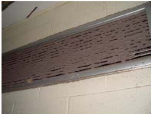
Figure 4: Main return grilles behind stage of cafetorium blocked b/c maintenance staff unaware of their locations.
