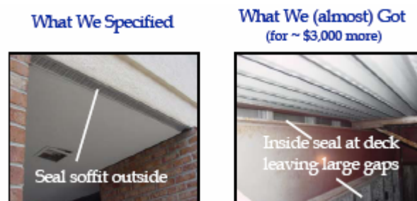
Figure 9: Specified vs. contractor planned soffit sealing solutions.
