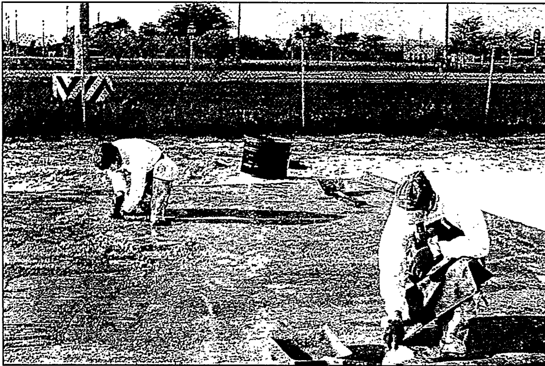
Figure 3. Concrete floor coating removal using PCRS-5.
