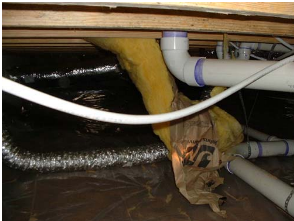
House address 104: Fallen batt and mold
