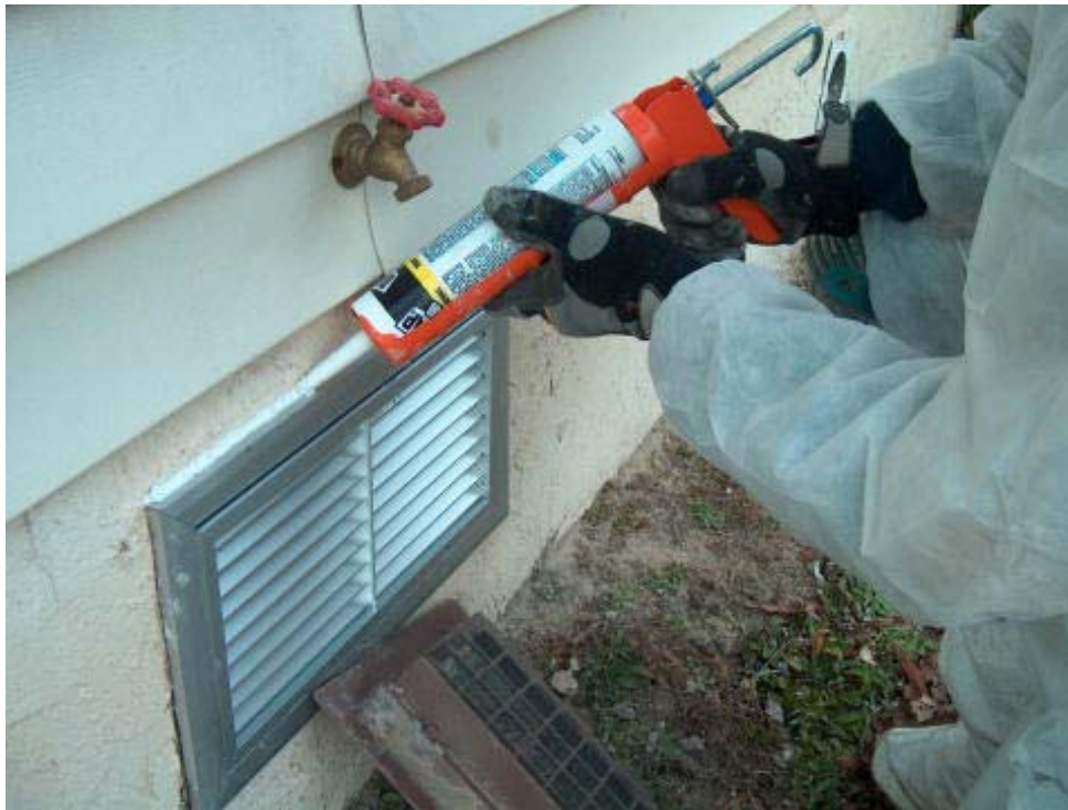
Sealing outside of ventilation intake to perimeter wall
