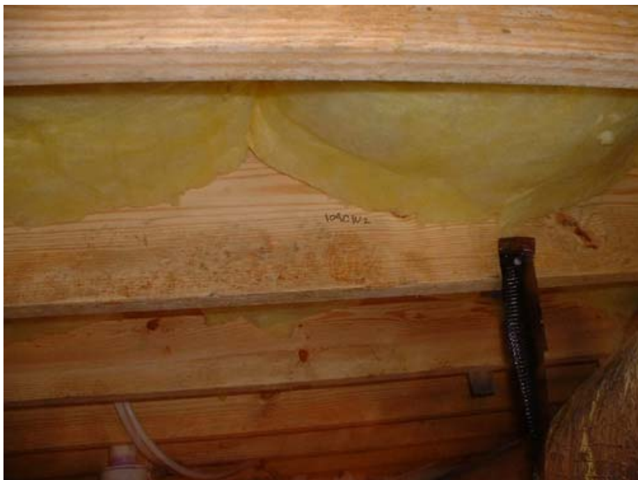
House address 104: Light red mold
