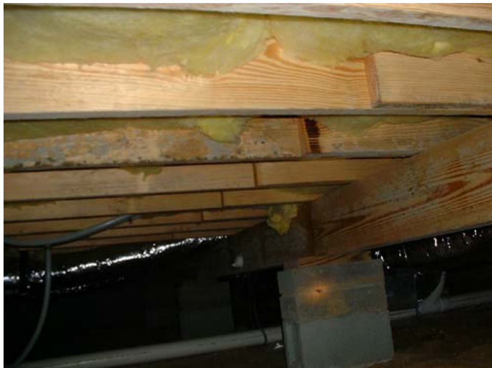
House address 107: Mold beam and joist
