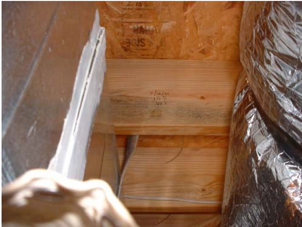
House address 100: Light mold
