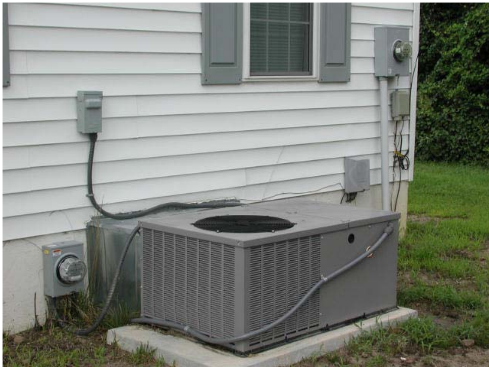
Sub-meter visible at left of duct cowling
