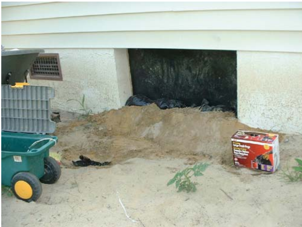
House address 110: Sandbagged access
