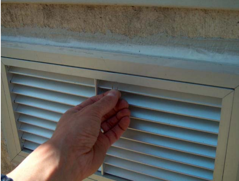
New ventilation intake opens without a tool
