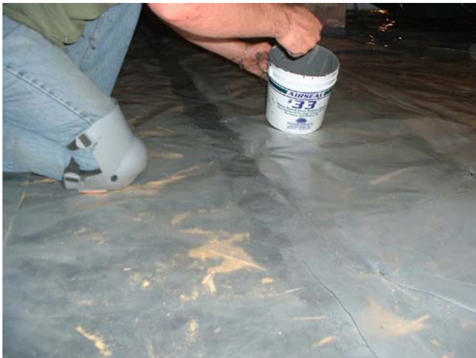
House address 106: Seal floor poly seams
