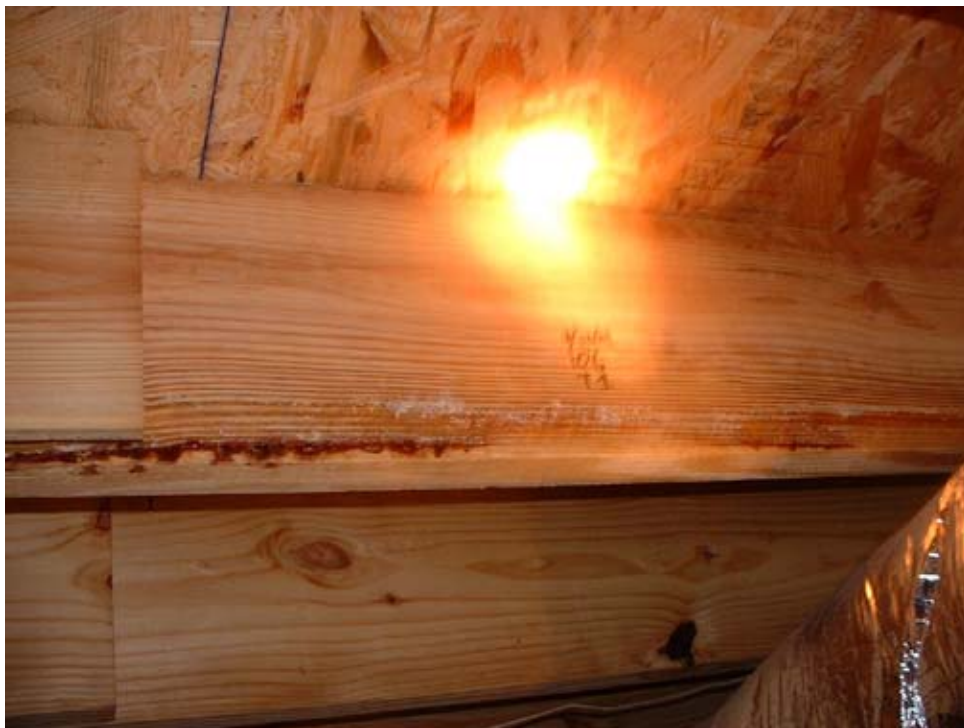
House address 106: Slight mold
