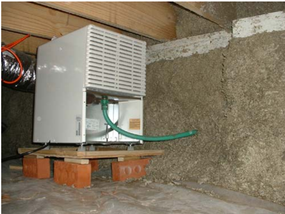
House address 109: Dehumidifier and wall insulation
