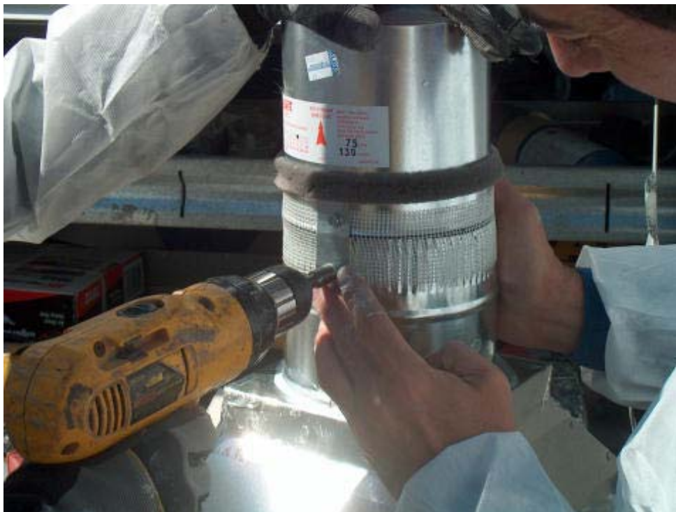
Attaching constant air flow regulator to new ventilation intake/filter
