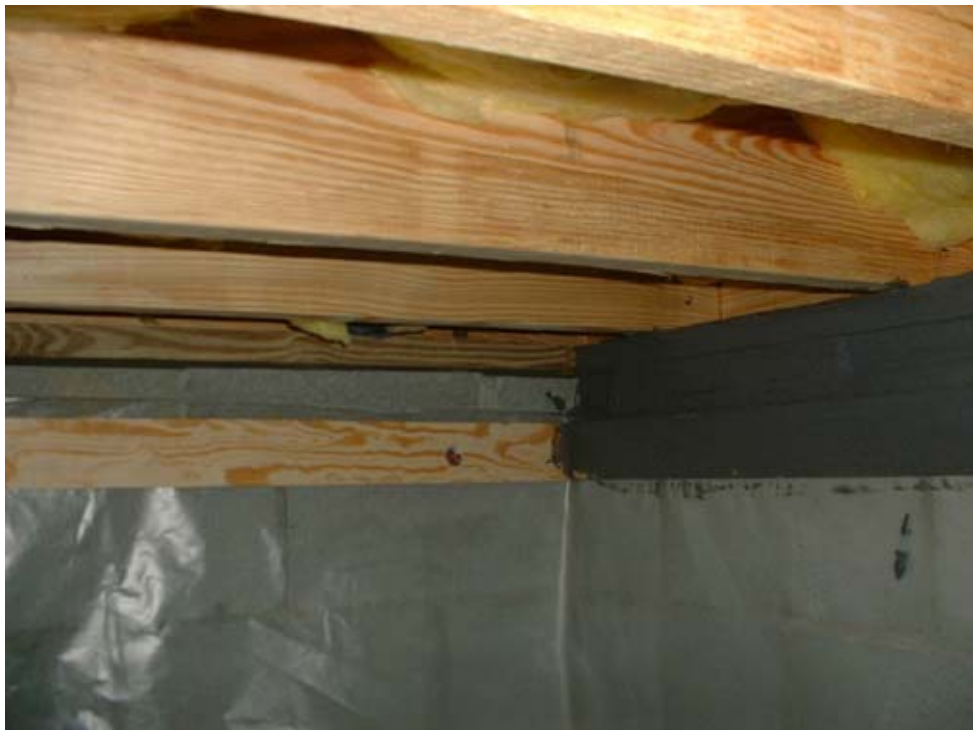
House address 106: Termite view strip and wall vapor barrier
