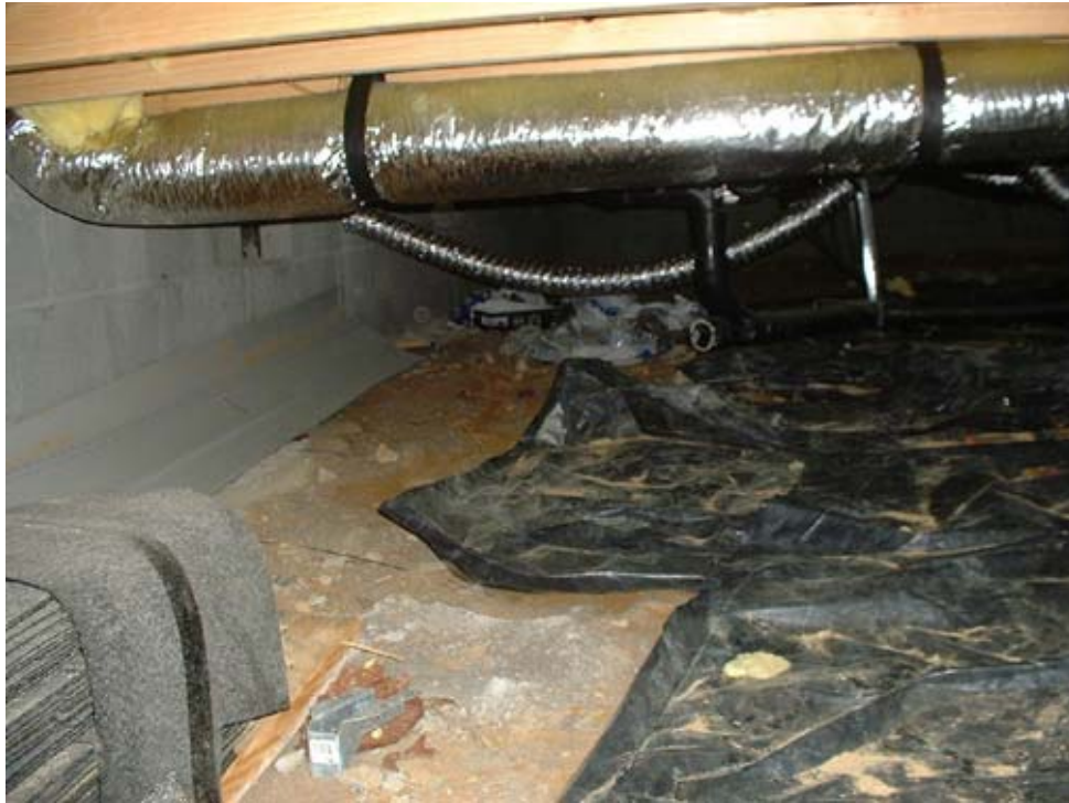
House address 100: No continuous vapor barrier
