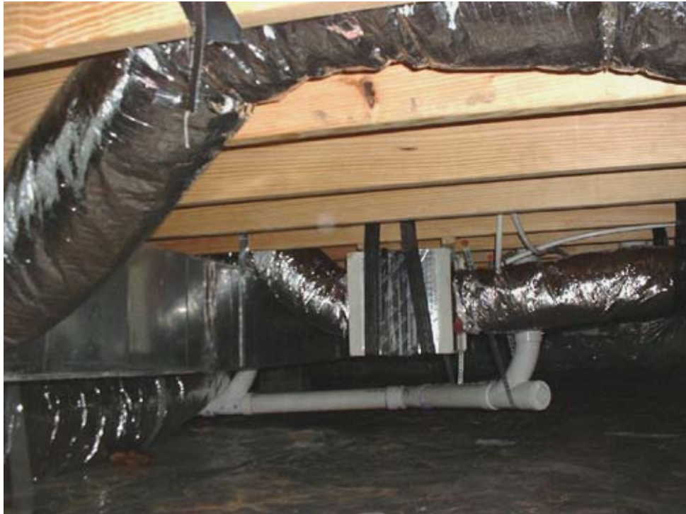
House address 105: Filter for ventilation system air – no mold on framing
