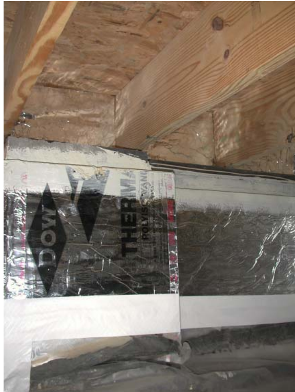
Wall-insulated closed crawl space, Phase II
