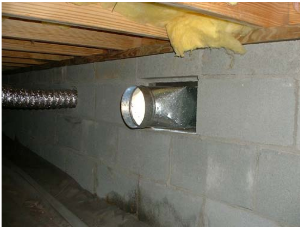
Transition installed in foundation
