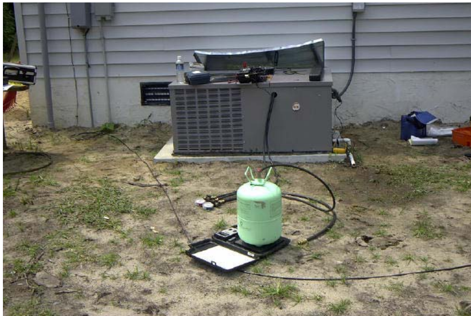
Checking heat pump refrigerant charge and air flow
