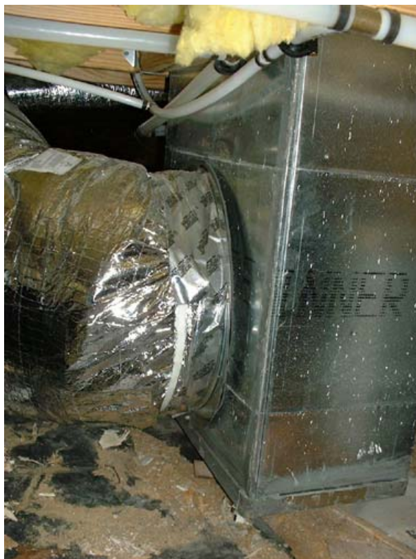
House address 106: Return duct air leakage
