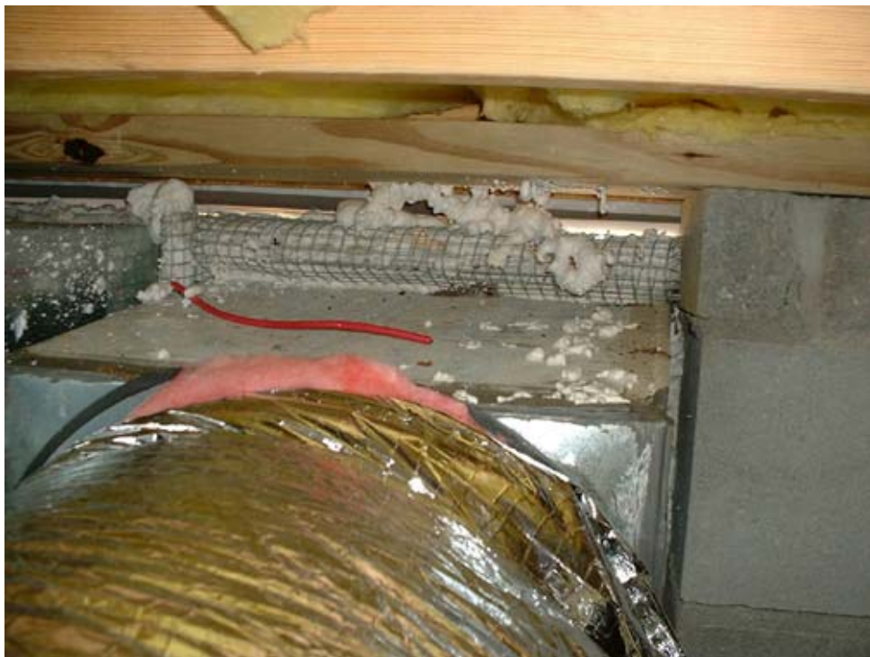
House address 103: Poor HVAC duct seal
