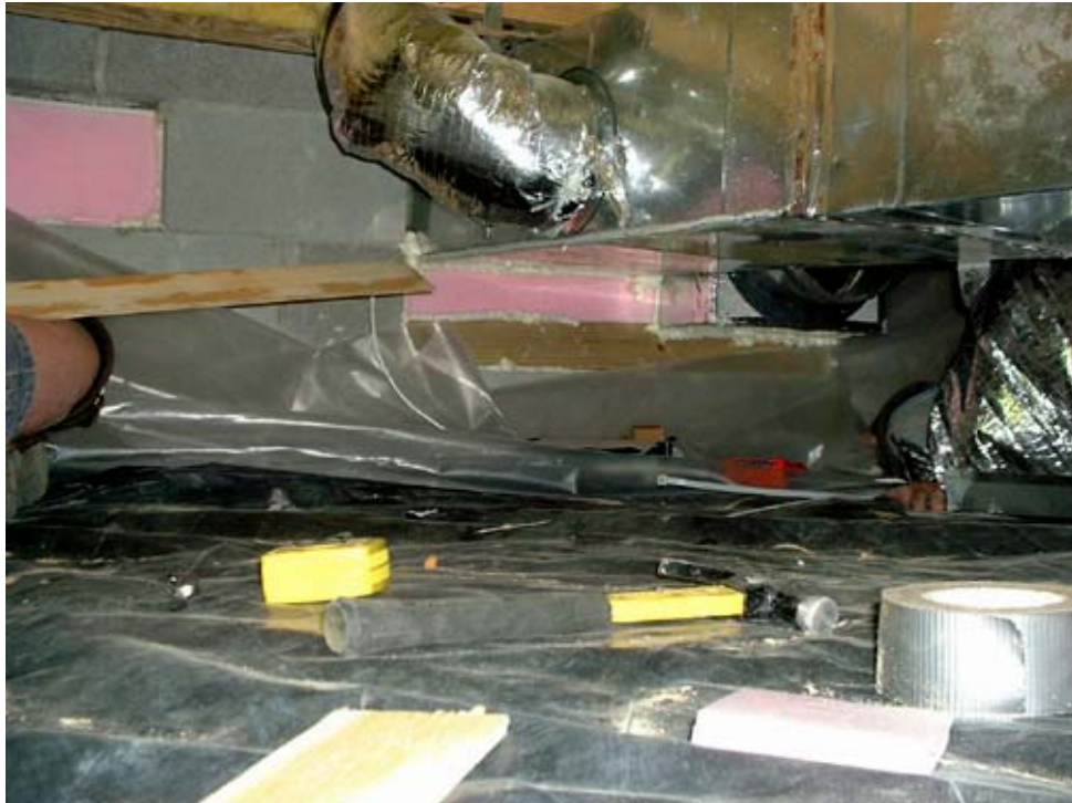
House address 106: Foundation vent and heat pump duct wall penetration sealing
