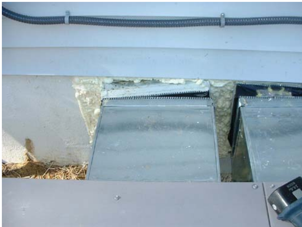
Heat pump duct crawl space wall penetration seal
