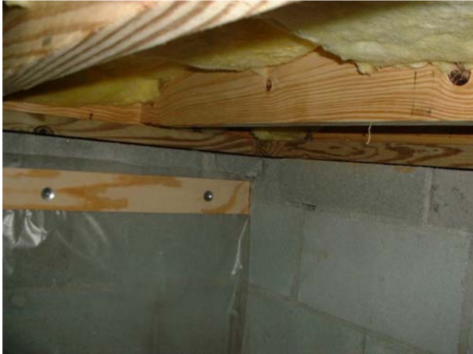
House address 106: Poly seal wall in progress
