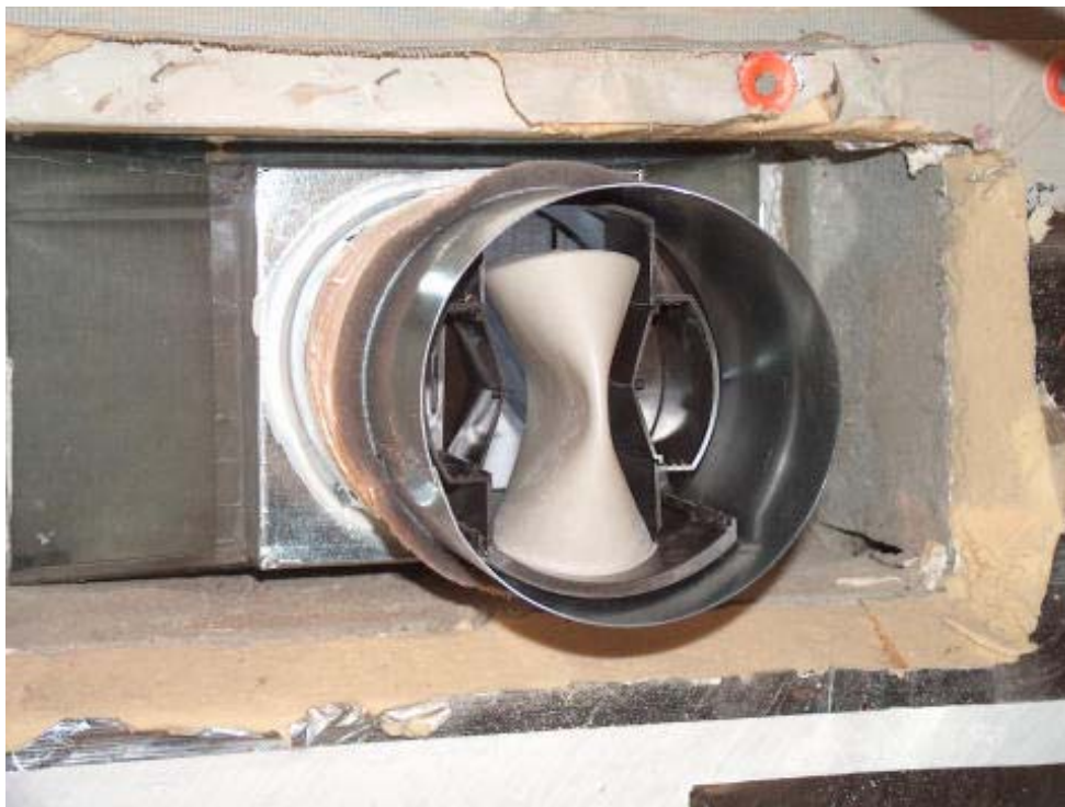
New intake assembly in old vent penetration, CAR visible
