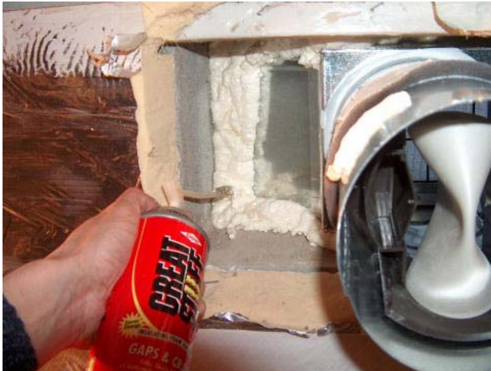
Sealing ventilation intake to perimeter wall
