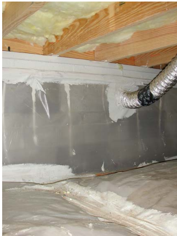
Floor-insulated closed crawl space, Phase II
