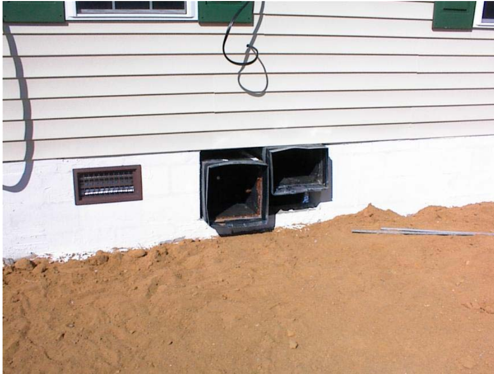
Return and supply ducts for package heat pump
