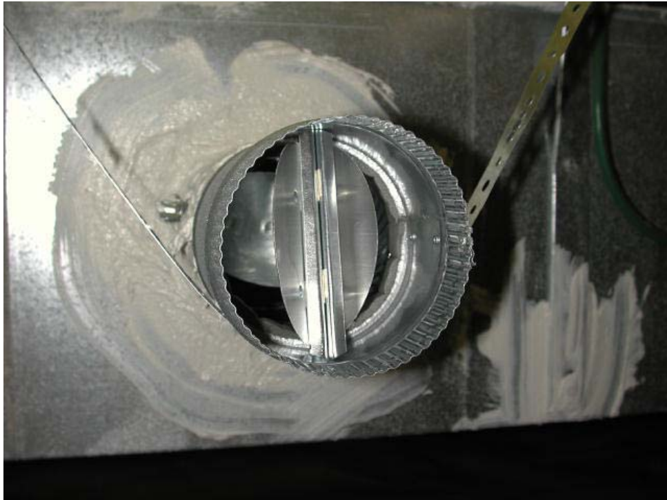
Balancing and butterfly dampers visible in well-supported crawl space supply duct
