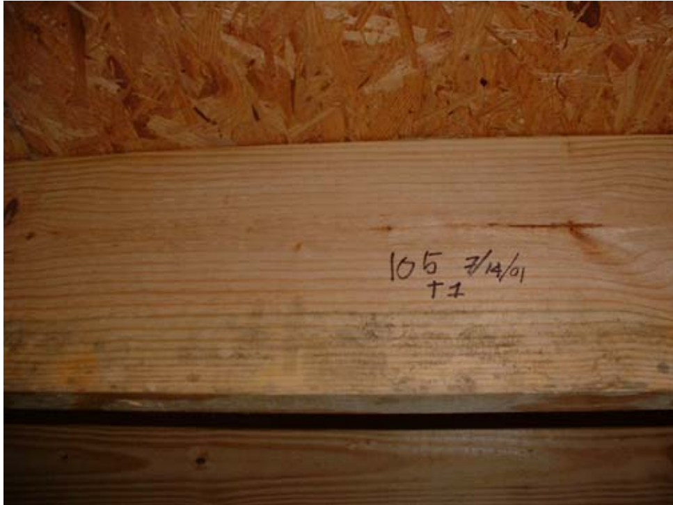
House address 105: Mold with labeling
