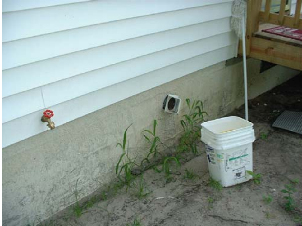
House address 107: Poor wall seal at dryer vent
