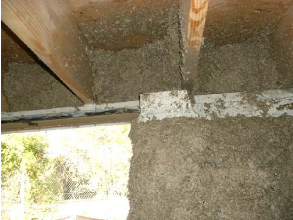
House address 109: Band joist and crawl space wall insulation
