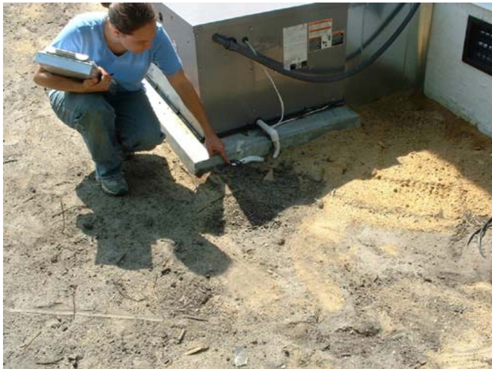
House address 104: Buried condensate drain
