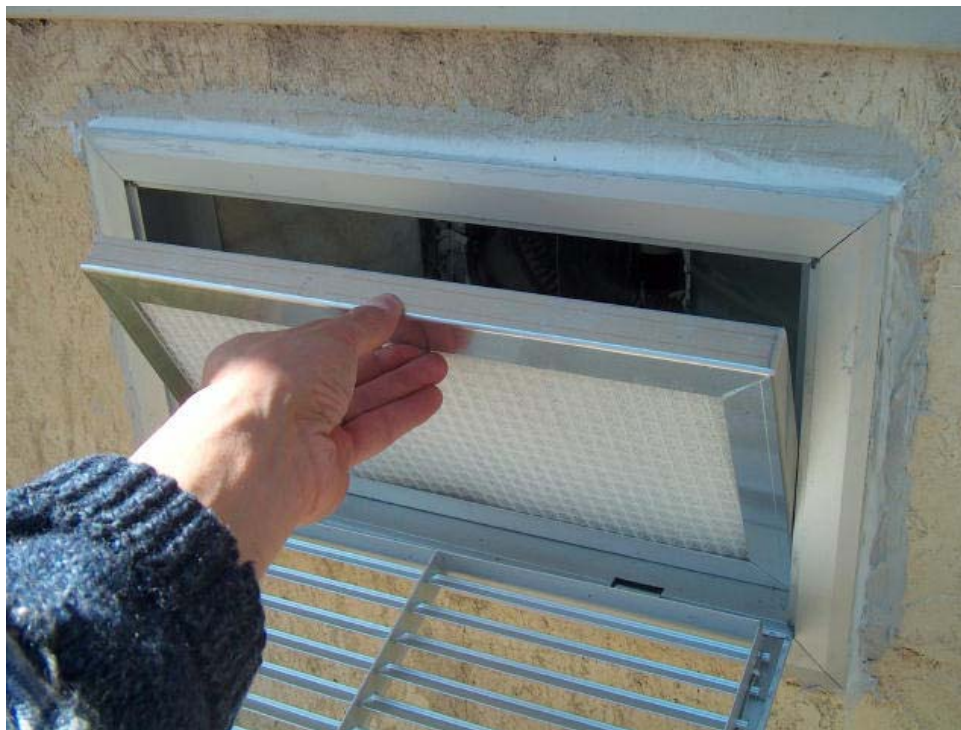
Filter behind the intake grill can be removed, washed, and reused
