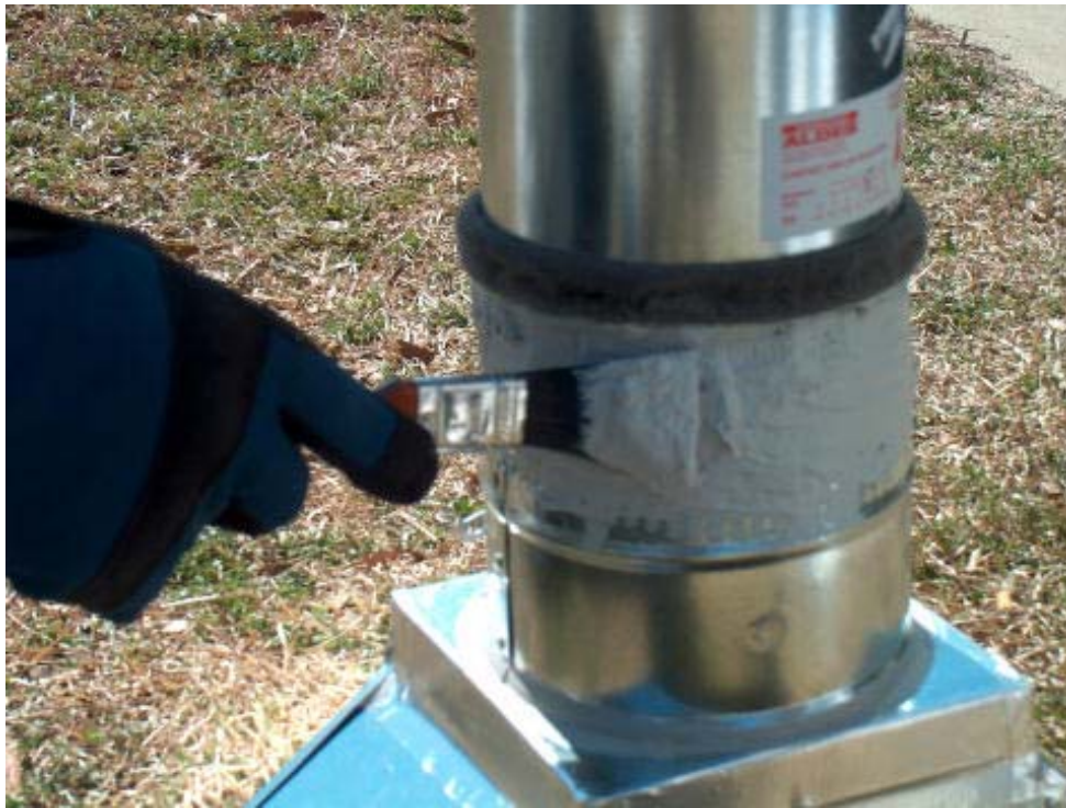
Sealing joint between CAR and ventilation intake with duct mastic
