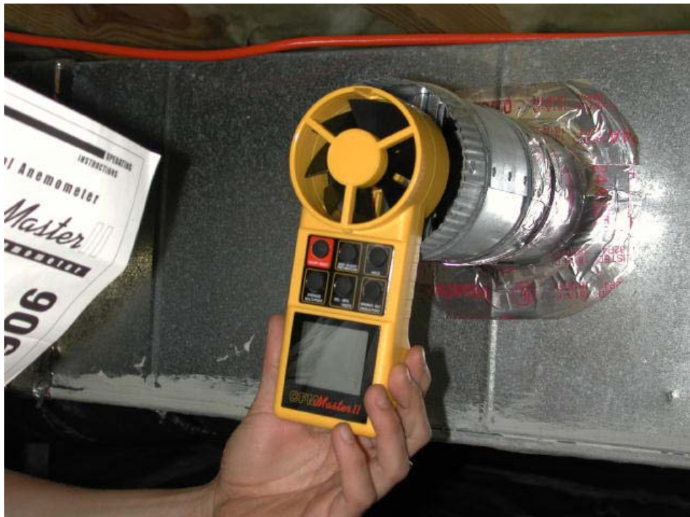
Taking velocity measurement reference to set remaining supplies
