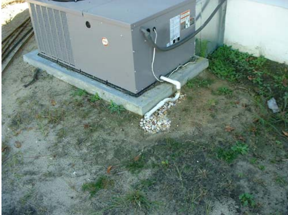
Heat pump condensate drain to gravel-filled pit
