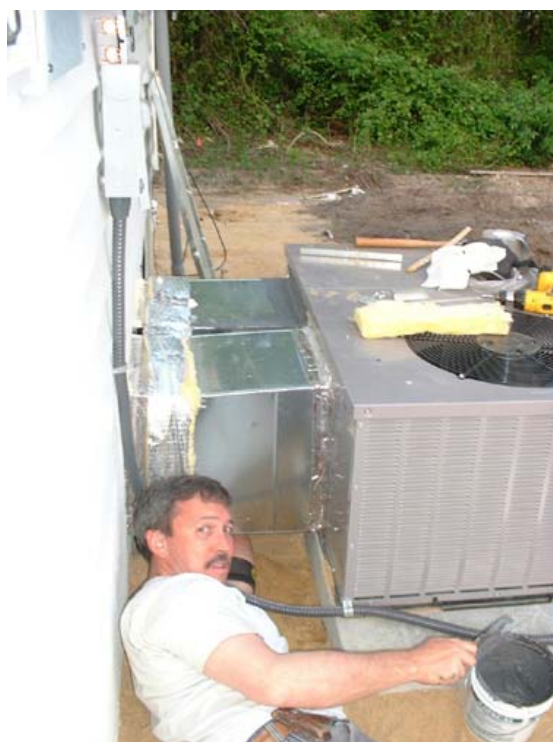
House address 106: Duct seal at package heat pump
