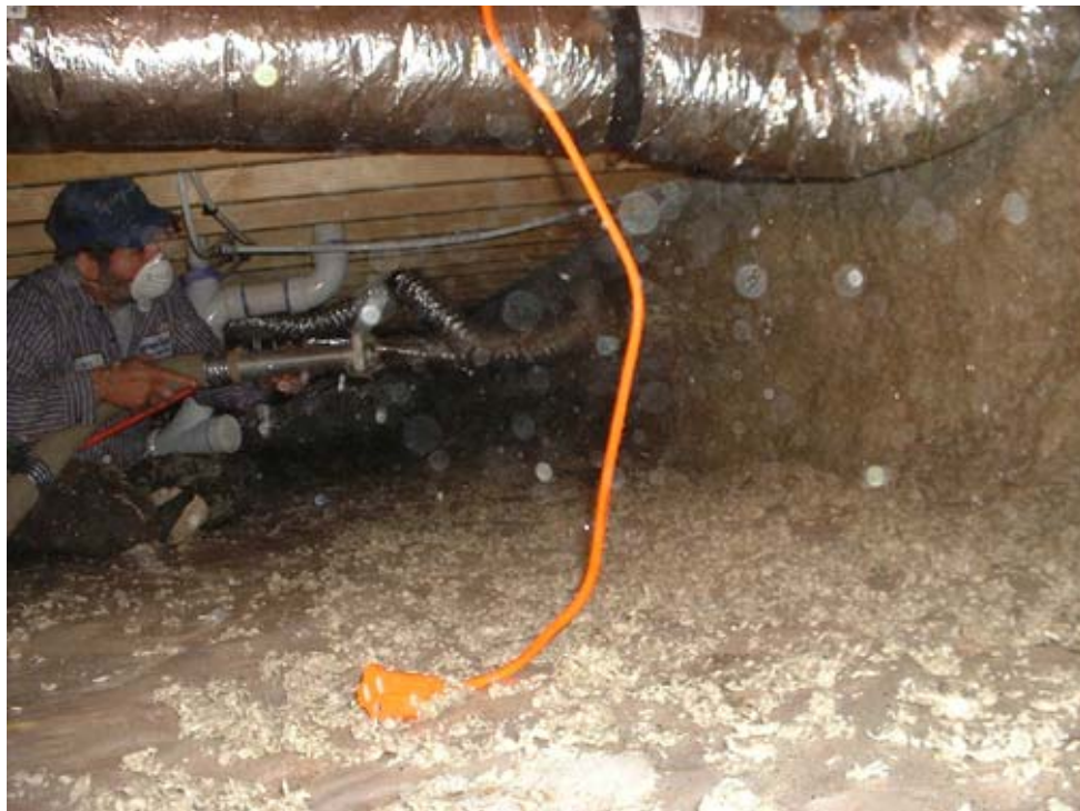
House address 109: Crawl space wall insulation
