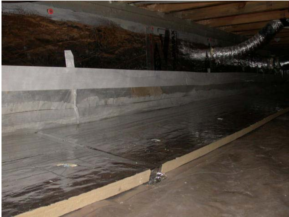
Horizontal ground insulation added to wall insulation for Phase IV
