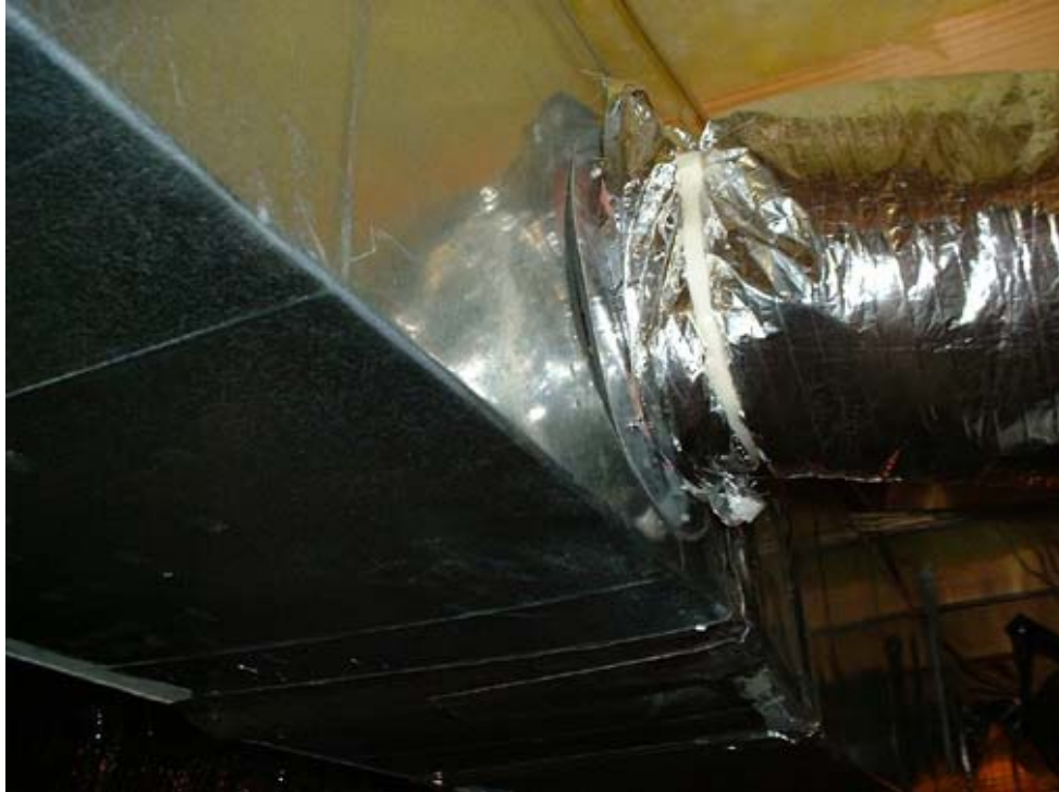
House address 110: Poor supply seal
