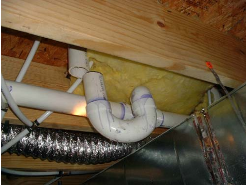
House address 111: Faulty plumbing trap at tub
