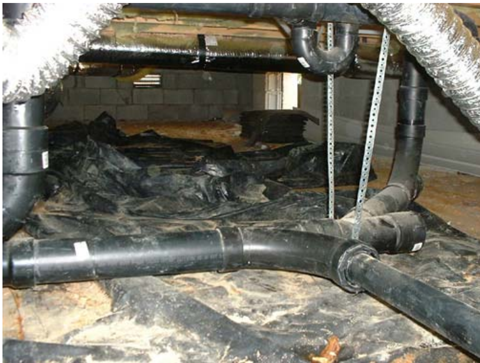
House address 100: No continuous vapor barrier
