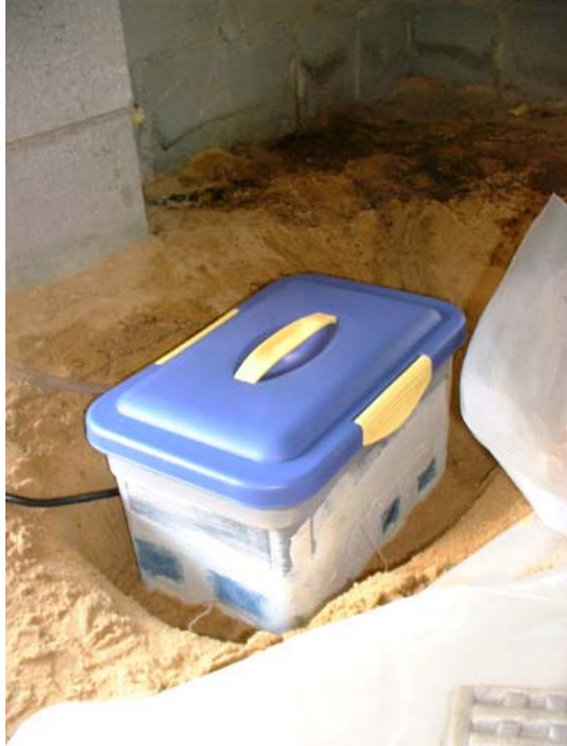
House address 110: Condensation sump pump – temporary until site grading completed
