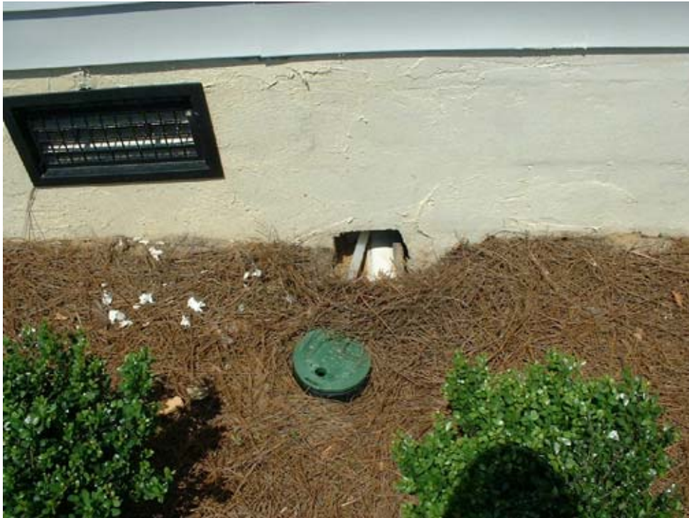
House address 111: Unsealed plumbing hole
