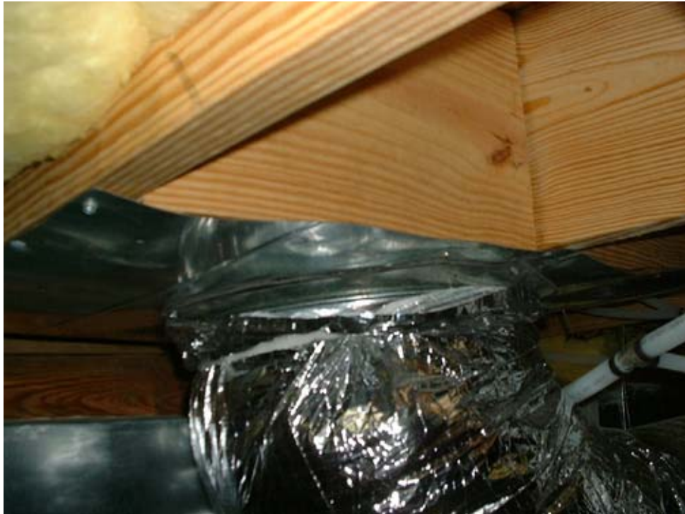
House address 100: Panned return air
