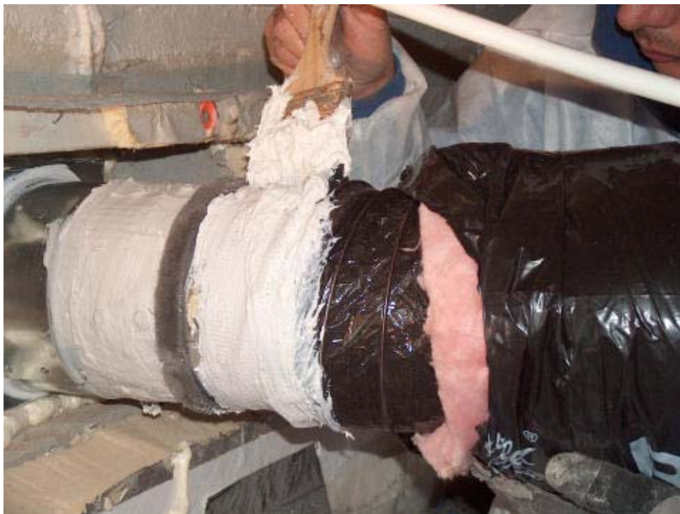
Sealing duct to ventilation intake with fiberglass mesh tape and duct mastic
