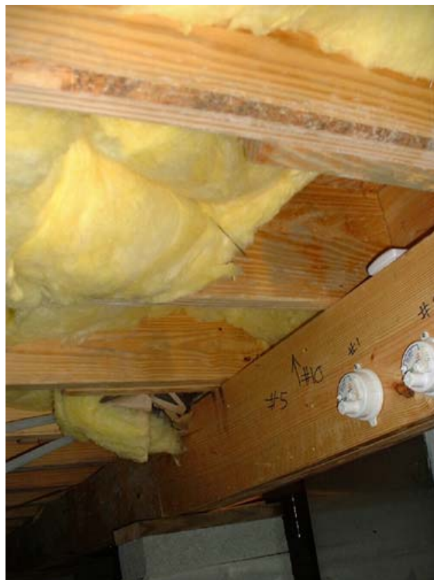
House address 110: Poor supply seal
