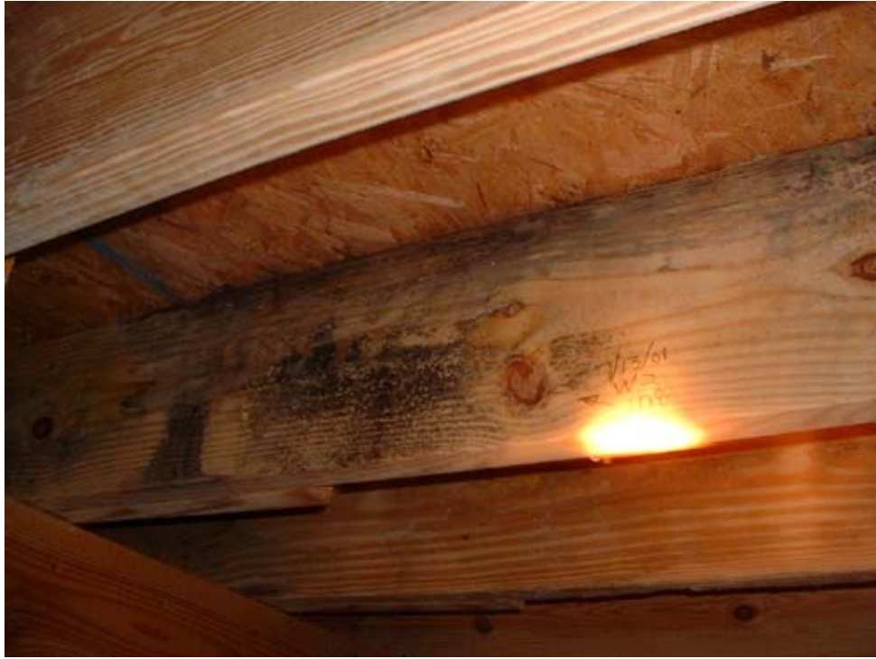
House address 108: Heavy mold
