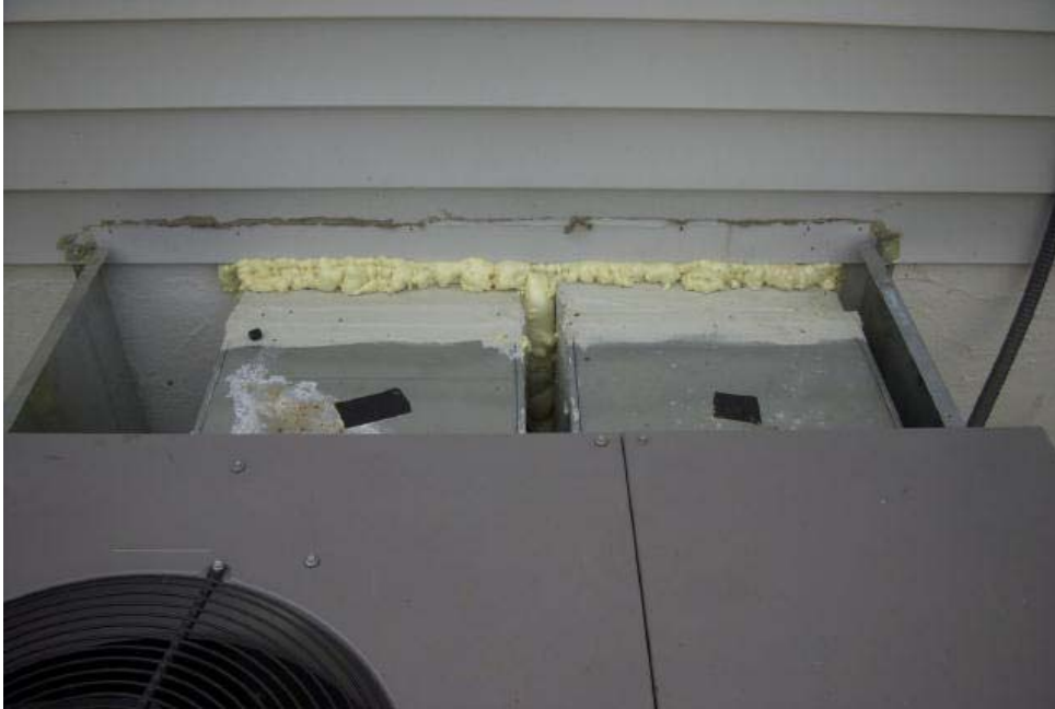
Sealed trunk ducts and package unit penetration
