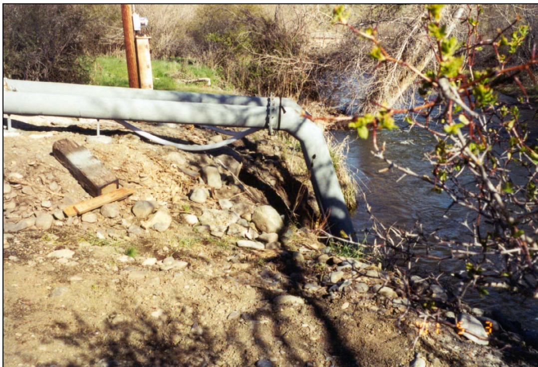
Photo 20. Suction Pipes from River to Pumps.
