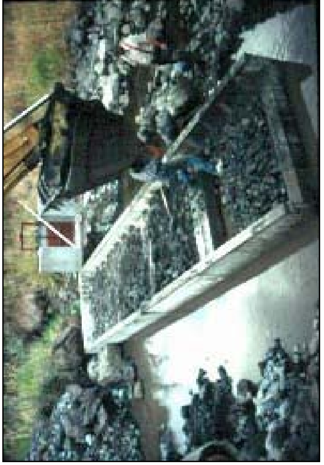
Photo 11. Filling Pre-cast Sill Boxes
