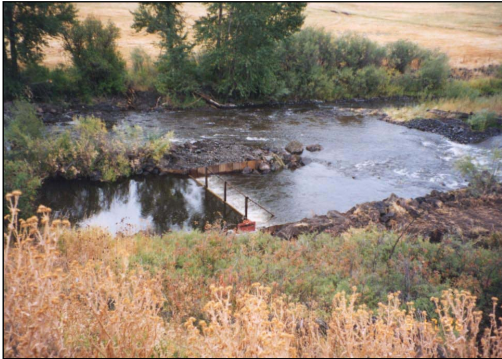
Photo 18. Typical permanent diversion, flashboards installed
