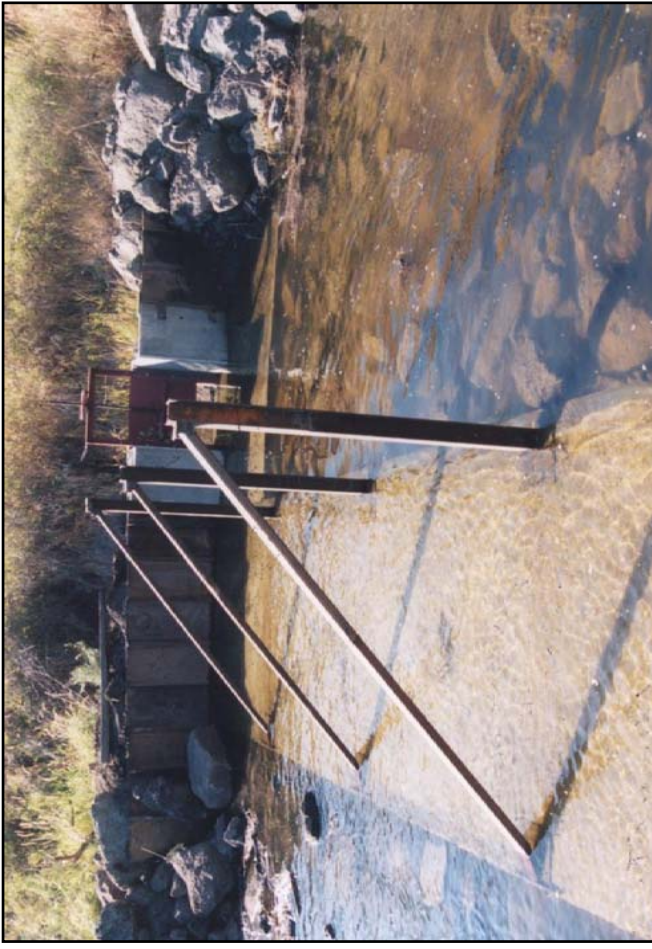
Photo 16. Typical permanent diversion, lay flat stanchions up, no flashboards
