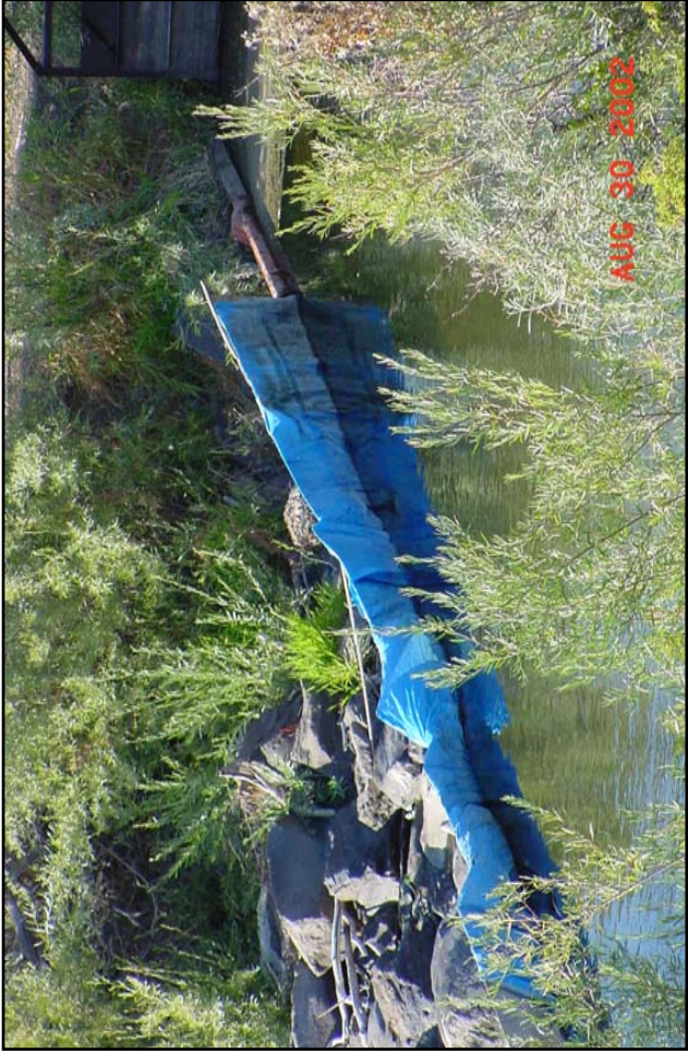
Photo 12. Typical gravel push-up diversion
