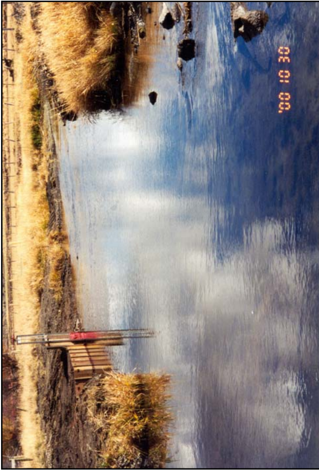
Photo 14. Typical permanent diversion, flashboards not installed
