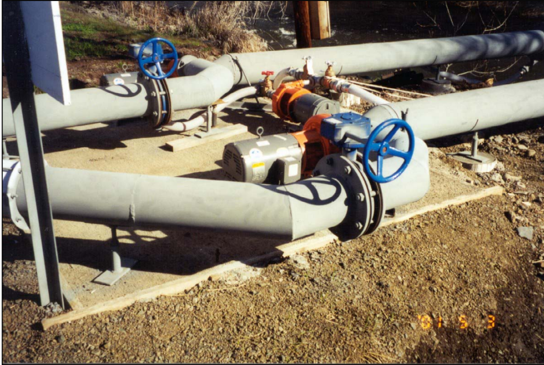
Photo 21. Turbine Pumps and Valves.
