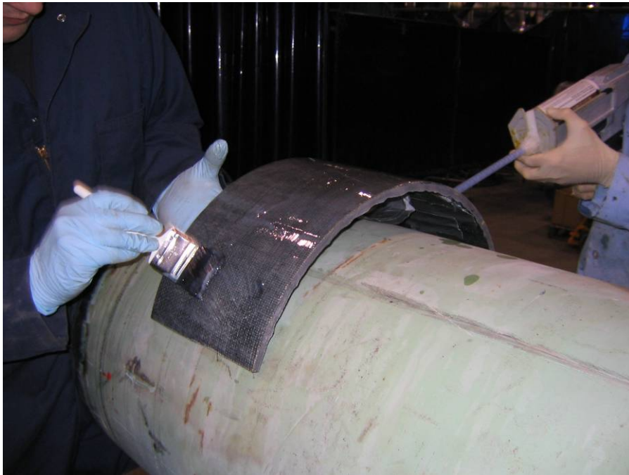
Figure 29 - Application of Adhesive to Repair Patch (Design 1)
