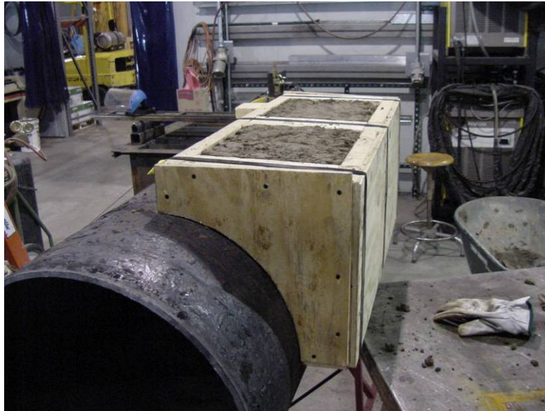
Figure 57 - Dirt Box for Weld Deposition Repair
