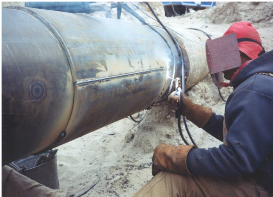
Figure 1 - Installation of a Full-Encirclement Repair Sleeve
