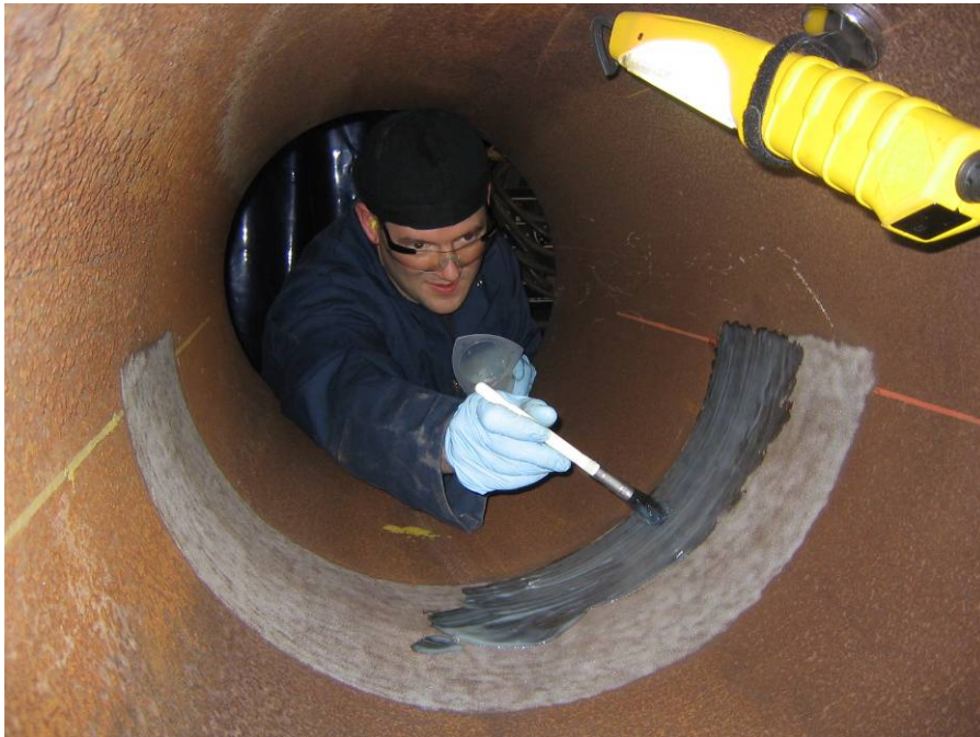
Figure 28 - Application of 3M DP460 Adhesive to Grit-Blasted Inside Diameter of Pipe
