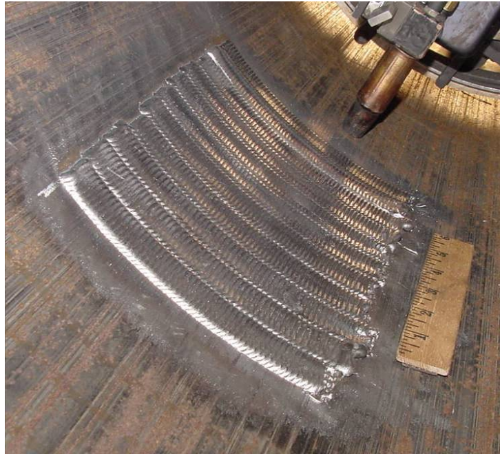
Figure 63 - Finished First Layer of Deposited Weld Metal on Inside Pipe Diameter
