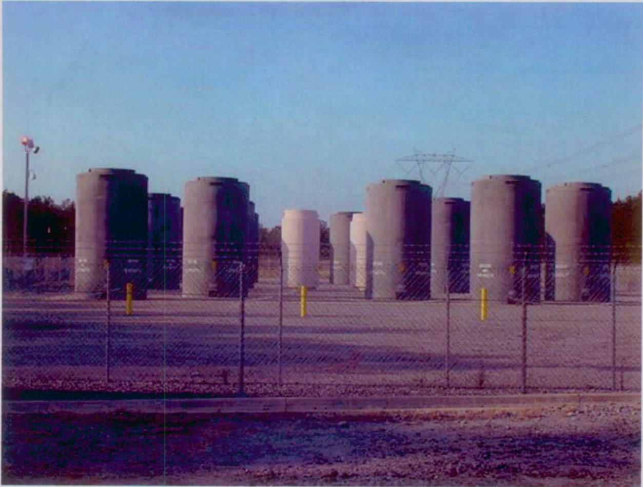
Figure B-8. Typical Concrete Site-Specific Cask for CSNF in Canisters
