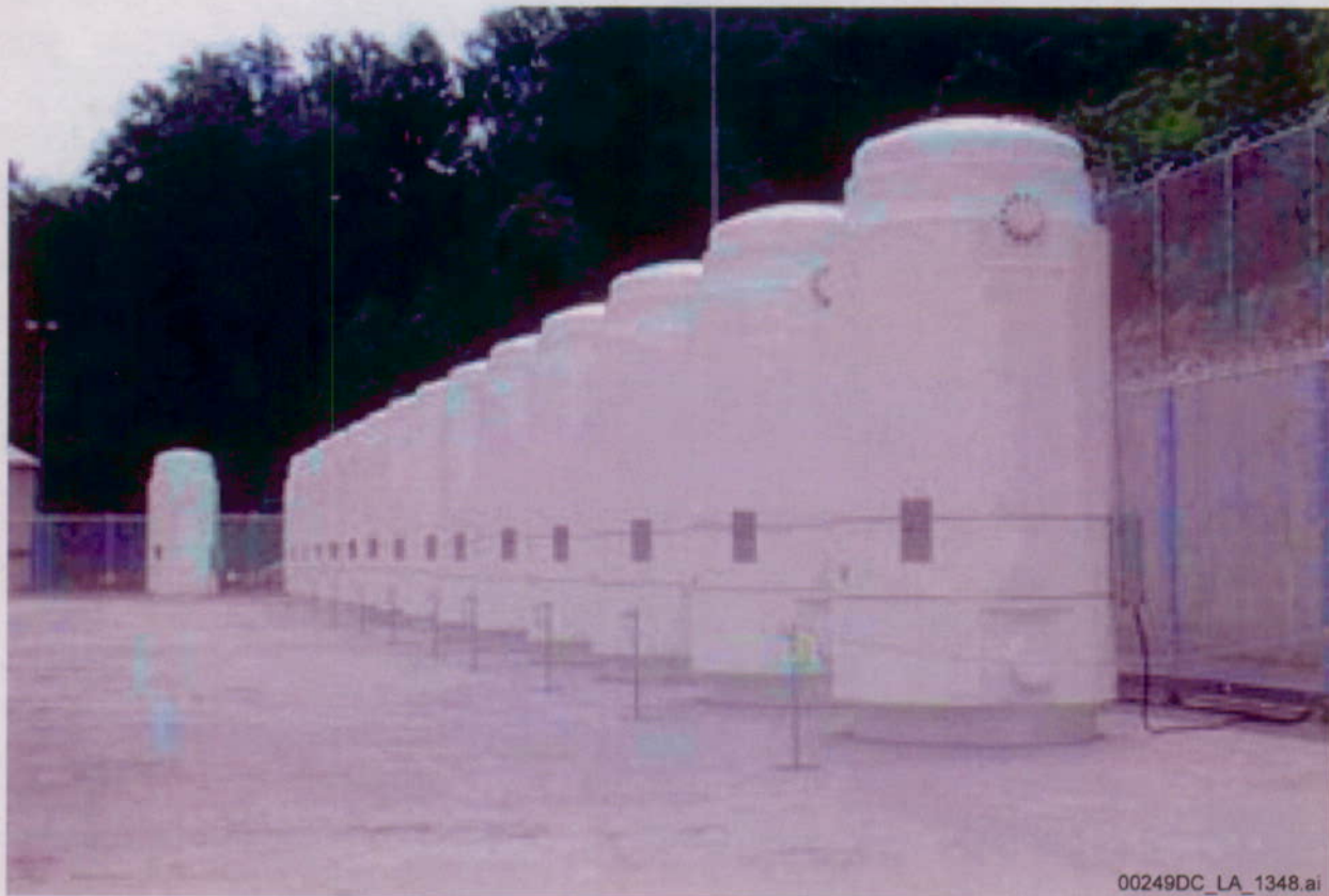
Figure B-9. Typical Metal Cask for Uncanistered CSNF
