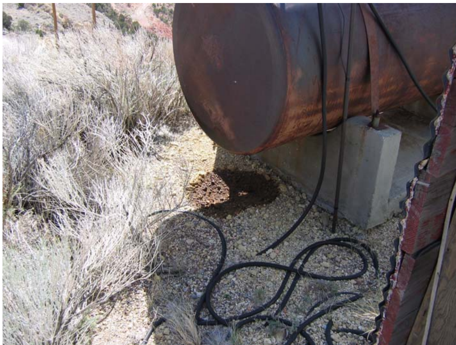
Figure A.1-5 Photograph of 550-Gallon Fuel Tank and Underlying Stain in CAU 551
