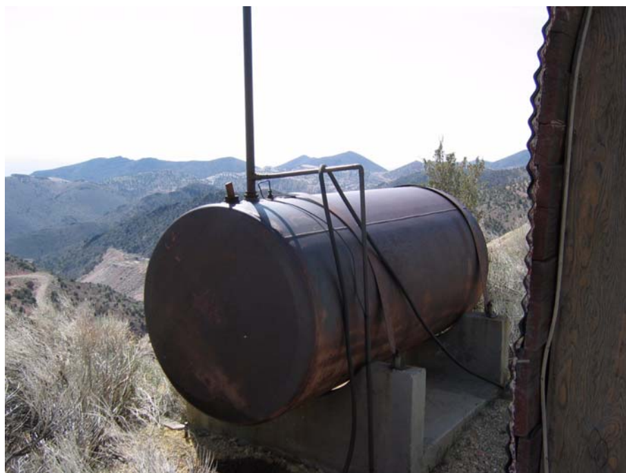
Figure A.1-4 Photograph of 550-Gallon Fuel Tank in CAU 551
