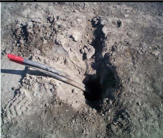
Borehole heat exchanger completion – grouting, spacing
