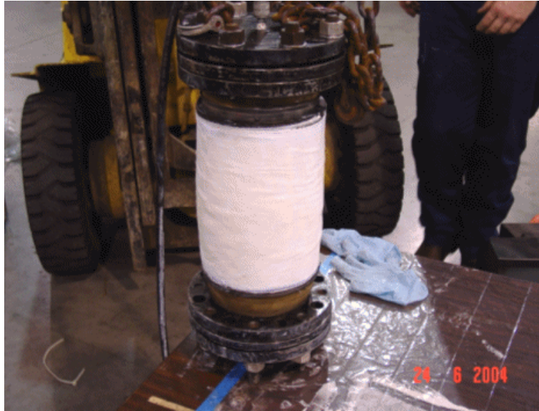
Figure 7. Repair Sleeve with Epoxy Applied
