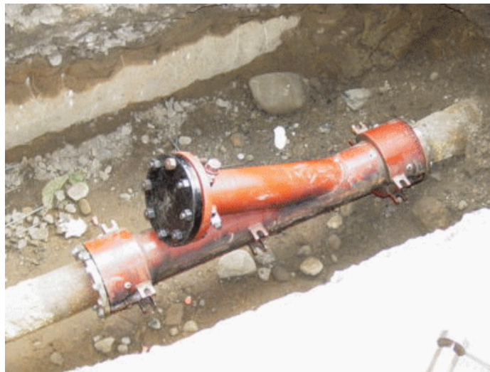
Figure 46. Entry Fitting Ready for Burial
