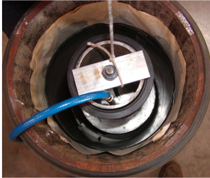
Figure 15. Bladder/Patch Assembly Hung in Joint
