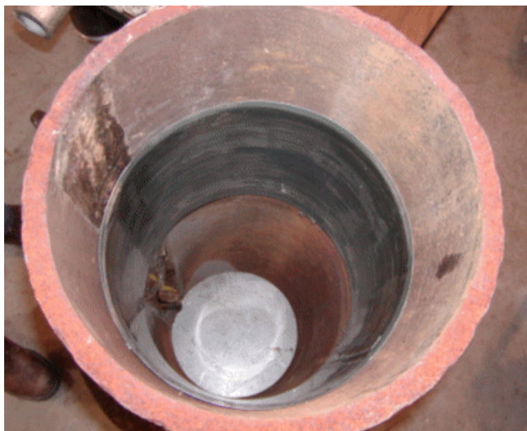
Figure 10. Successfully Installed Repair Sleeve
