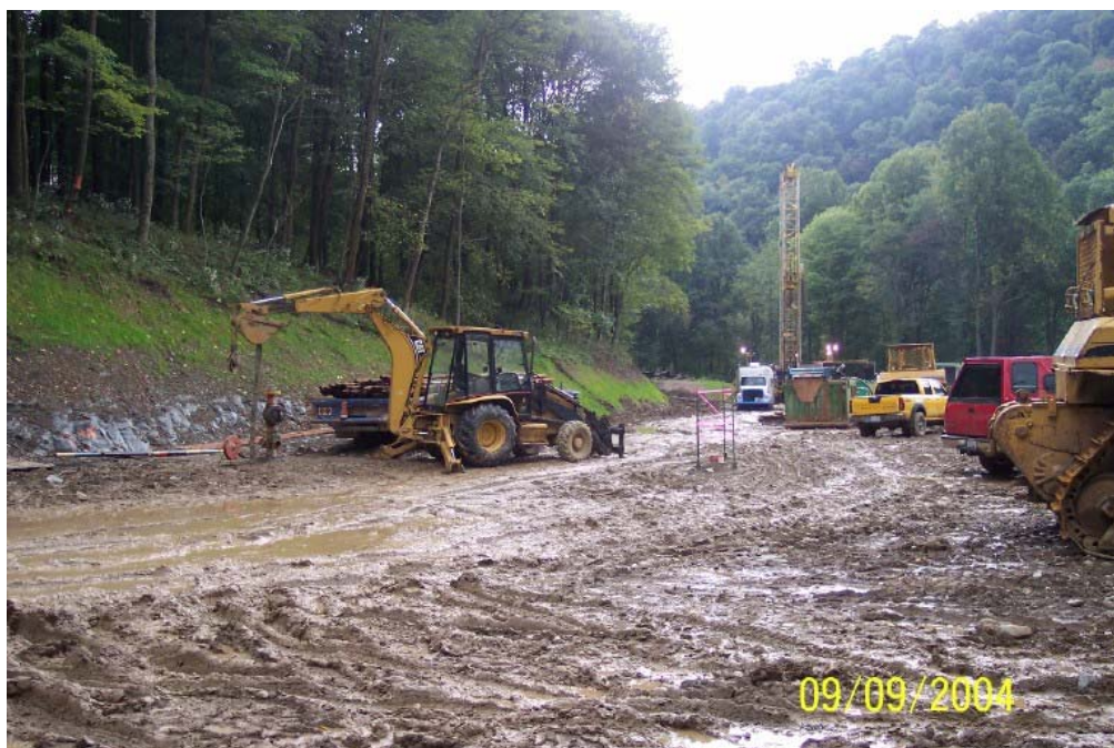
Figure 8: Center Site Upper Freeport Seam Drilling Activities with Vertical Well in Foreground and Access Well in Background – September 9, 2004
