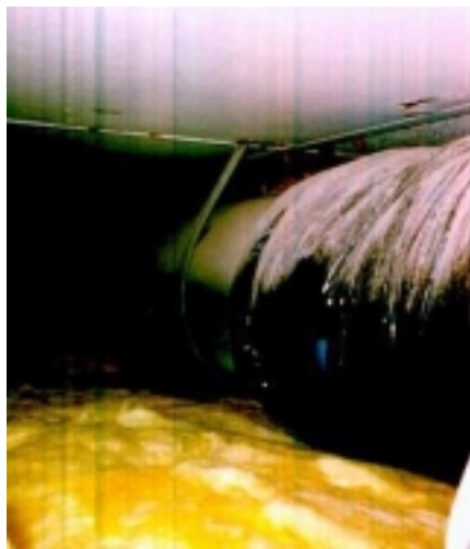
Figure 1.1.2: Drugstore ductwork installed above insulated ceiling tiles
