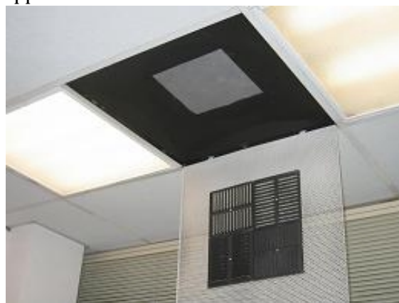
Figure 2.2.2: Foam plug in the central discharge of a hinged diffuser.
