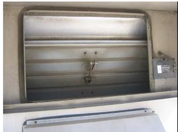
Figure 2.8.2: Damper and sensor module
