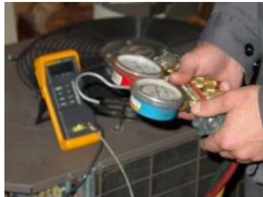
Figure 2.4.4: Measuring refrigerant pressures
