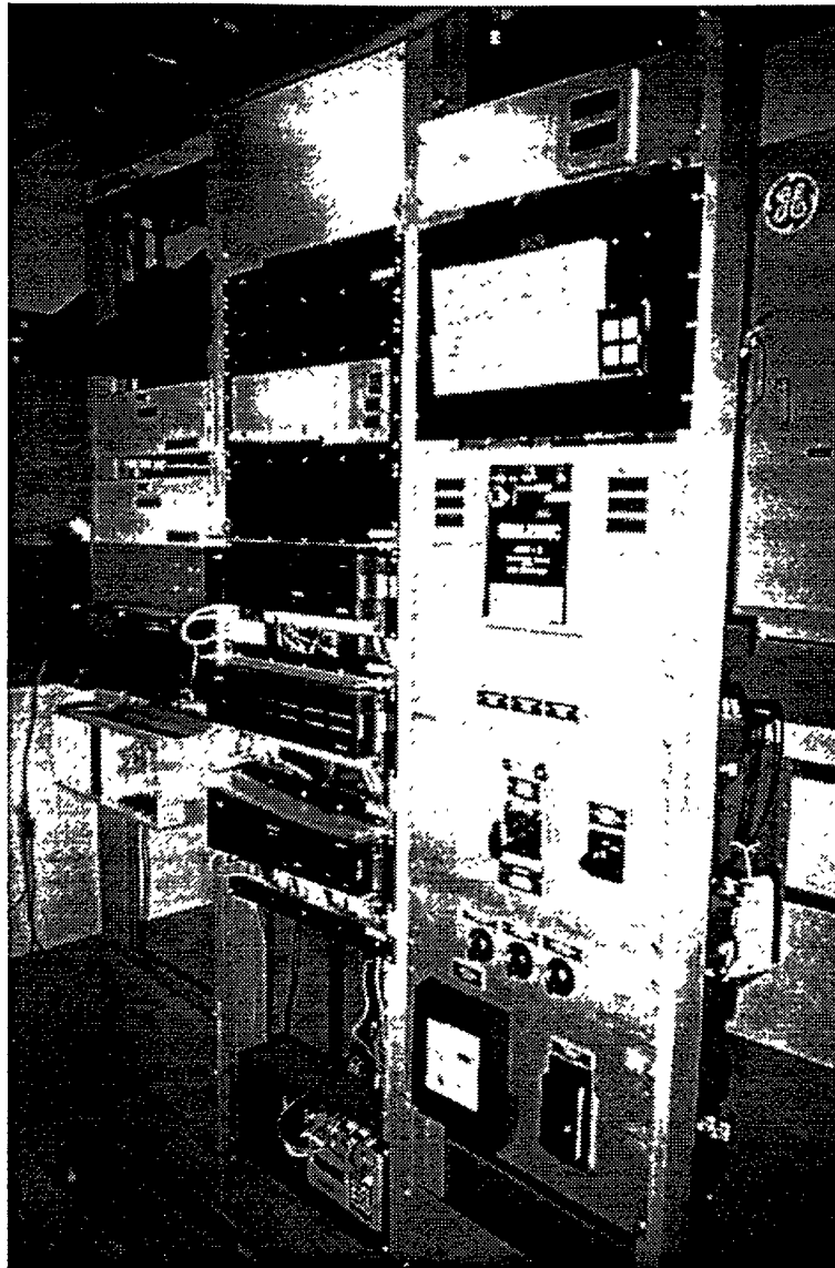
Figure 5-4. Kerman telecommunications, SCADA, and control racks (left to right).
