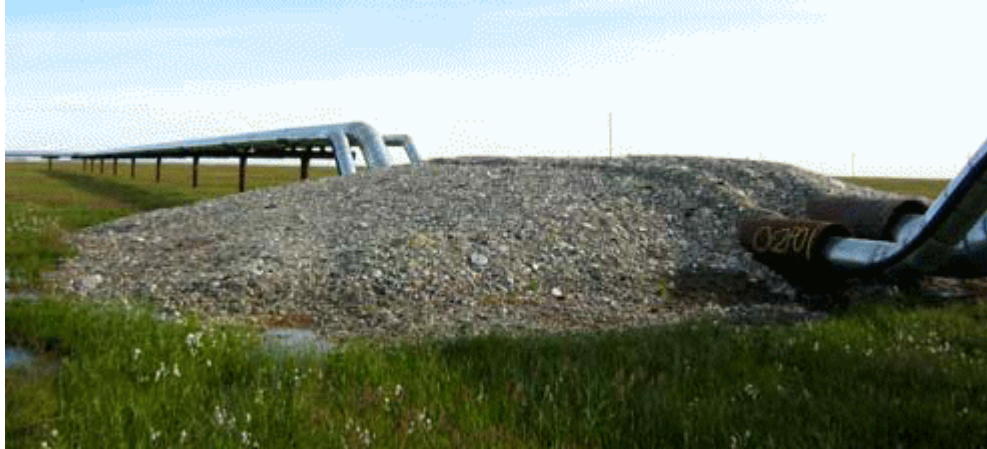
Figure 8. Gravel Ramp for Pipeline Crossing
