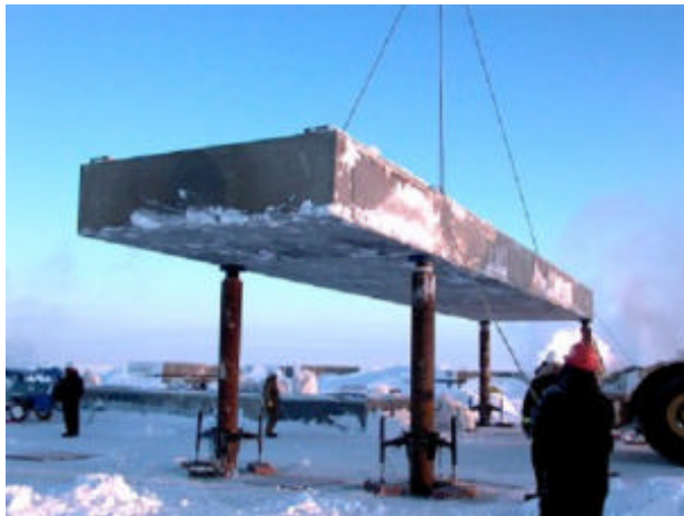
Figure A-3. Setting the First Platform Module
