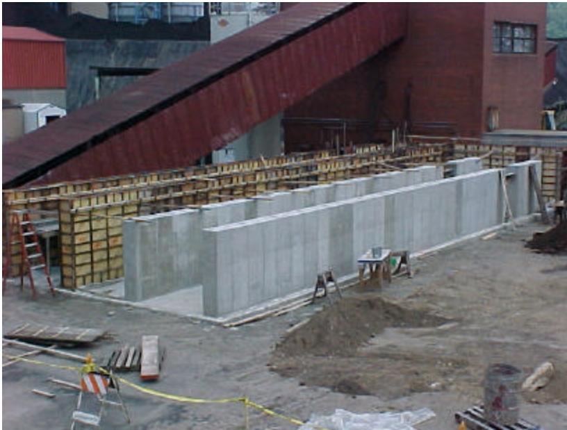
Figure 5-16. Construction of the foundation and support walls for the walking-floor bin
