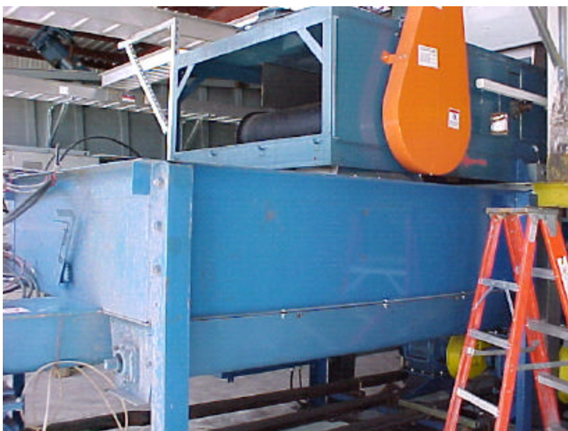
Figure 7-8. Installing the weigh belt feeder and live bottom bin at the Albright demonstration
