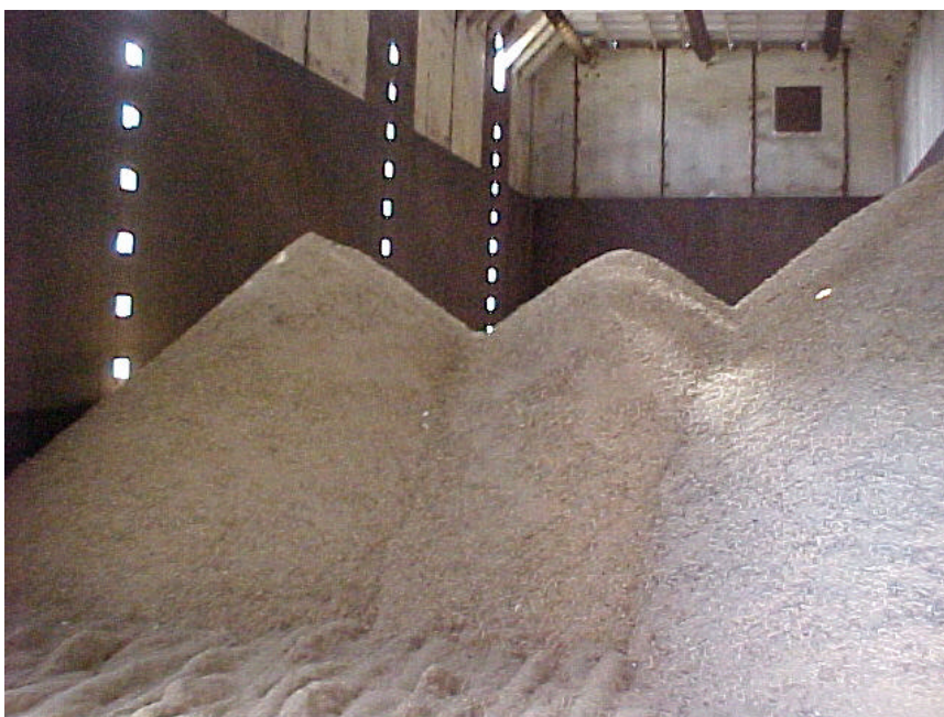
Figure 6-7. The walking floor bin receiving sawdust from the processing facility
