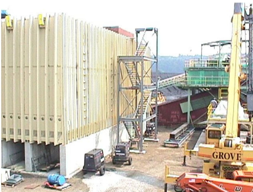
Figure 5-18. Construction of the walking floor bin walls
