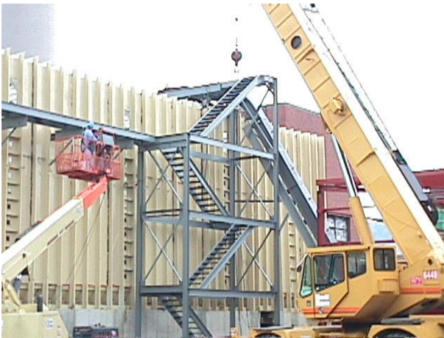
Figure 5-17. Construction of the walking floor bin
