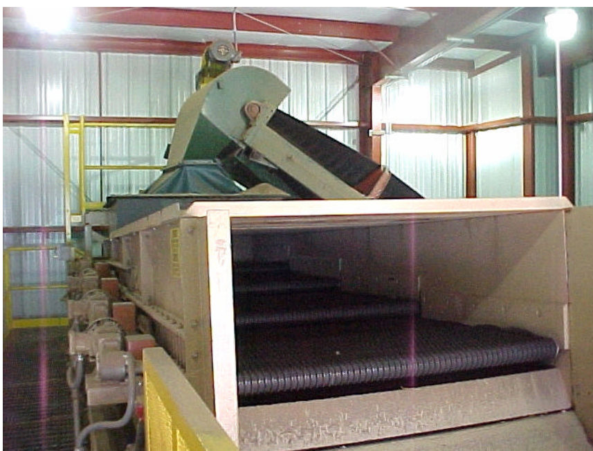
Figure 6-5. The disc screen installed at Willow Island Generating Station
