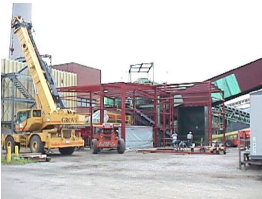
Figure 5-15. Construction of the processing facility including the sawdust receiving hopper
