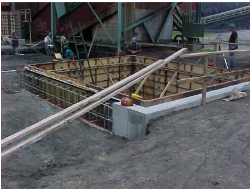
Figure 5-11. Construction of the fuel receiving pit, setting forms
