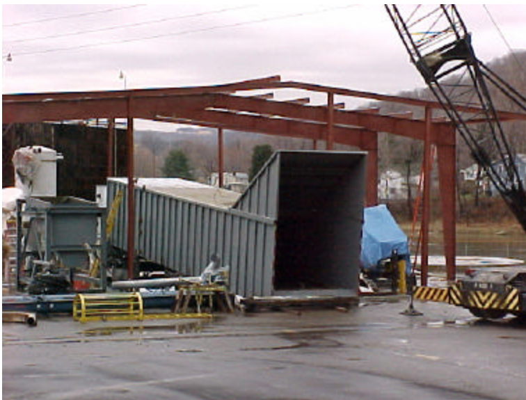
Figure 7-5. Framing the Albright building—front view featuring walking floor unloader
