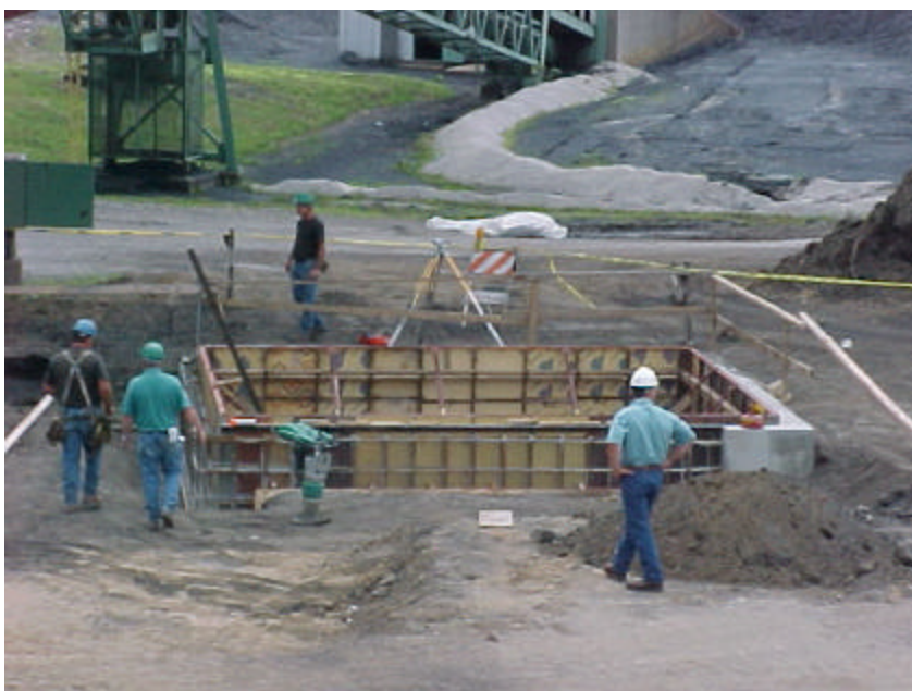
Figure 5-10. Construction of the fuel receiving pit
