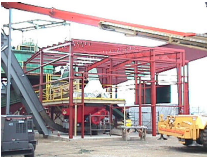
Figure 5-14. Construction of the processing facility including the disc screen, grinder, and outfeed conveyor
