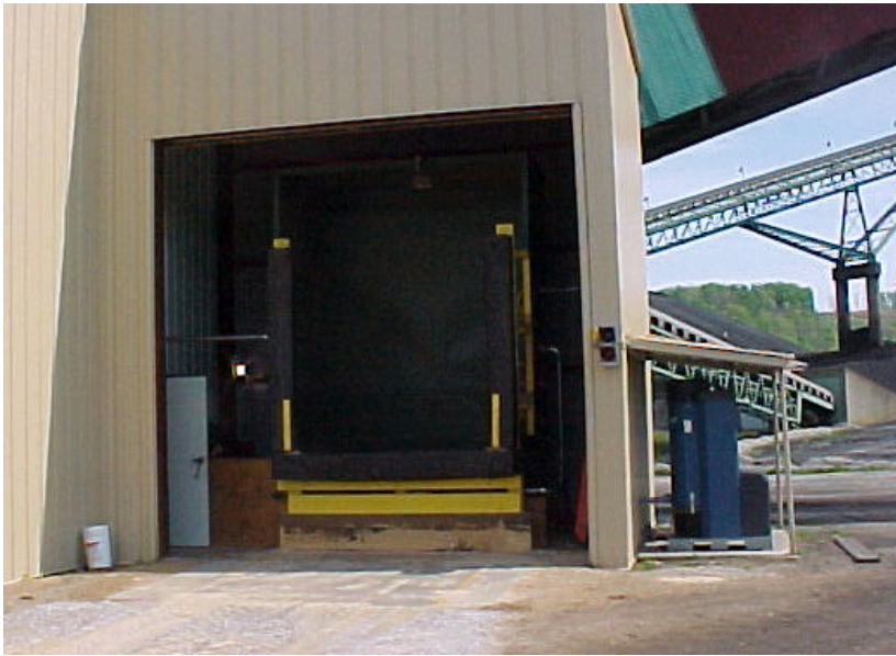
Figure 6-2. The sawdust receiving hopper and door. Note the vacuum system at the far right of the structure. This facilitates housekeeping and discharges captured sawdust in the receiving hopper
