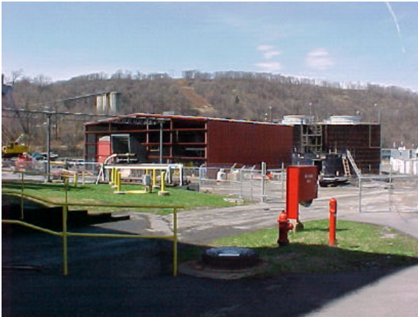
Figure 7-6. The Albright building partially enclosed, with the silo construction started (to the right of the building)
