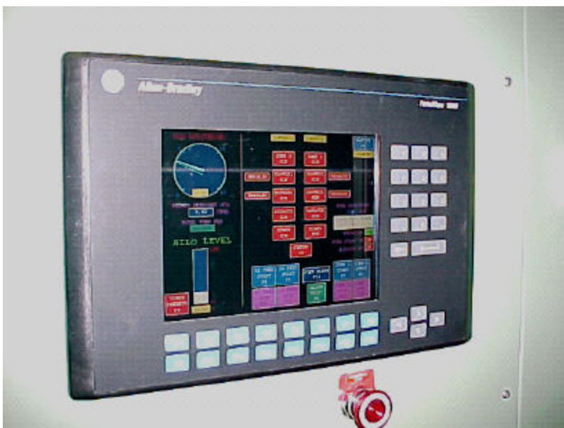
Figure 7-9. The control panel installed for the boiler operator at Albright Generating Station. Note the emergency stop just below the panel.
