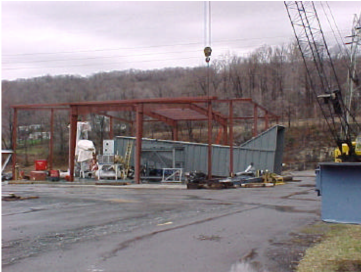
Figure 7-4. Framing the Building for the Albright Demonstration. Note the walking floor unloader already in place.
