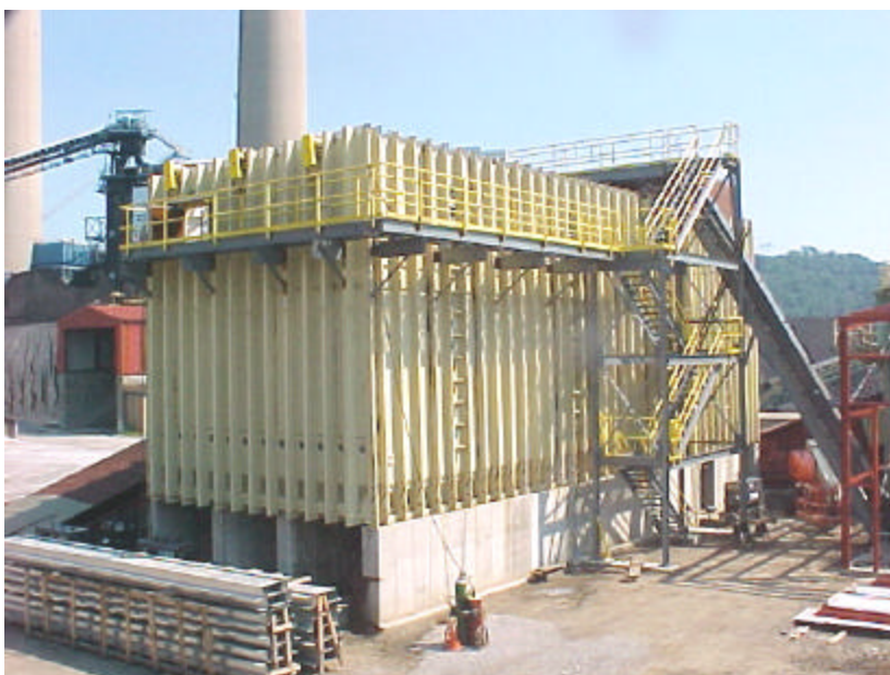
Figure 5-19. Completion of the walking floor bin and associated conveyor from the processing facility (under construction at extreme right)
