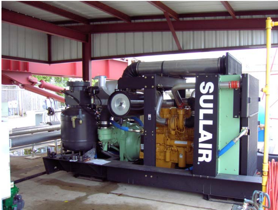
Fig. 3.61 New Sullair air compressor
