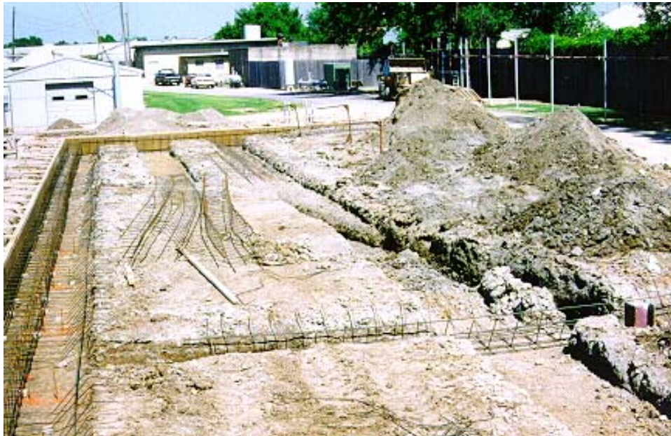
Fig. 3.6 Reinforcing steel
