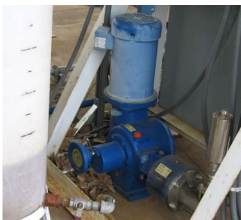
Fig. 12.7 Surfactant injection metering pump
