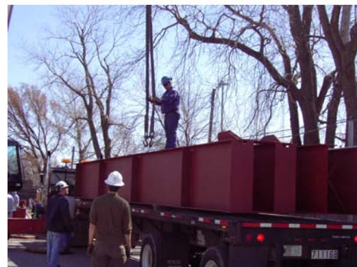
Fig. 3.48 Delivered mast pieces
