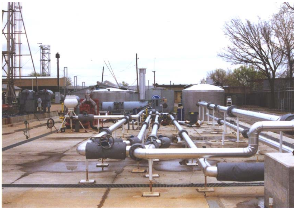
Fig. 3.17 Piping insulation
