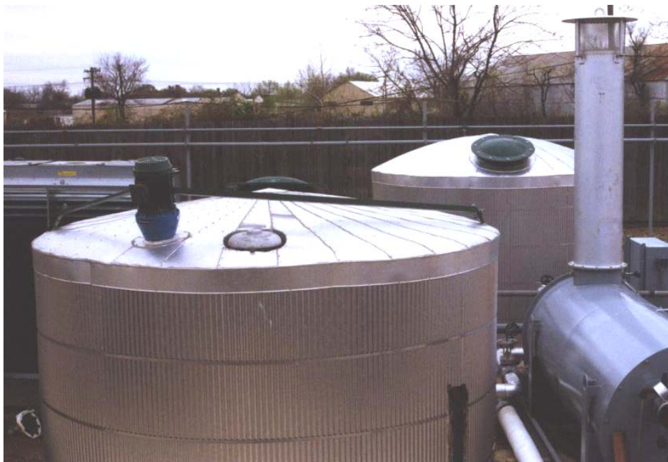
Fig. 3.16 Tank insulation
