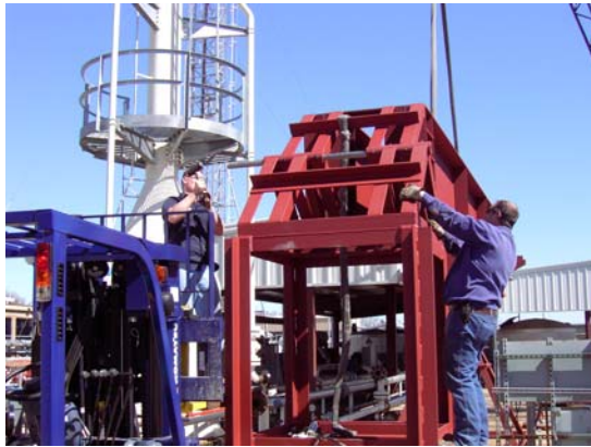
Fig. 3.49 Assembling of a hinged joint
