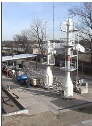
Fig. 3.32 Injection and removal towers after installation
