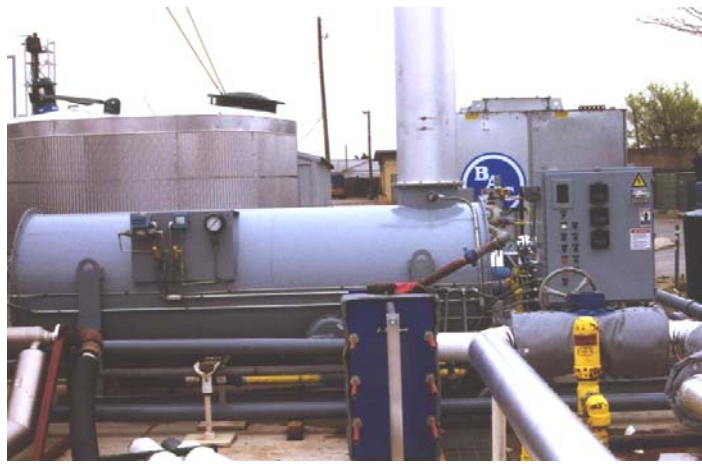
Fig. 3.13 Indirect fired boiler (2 mm BTU)
