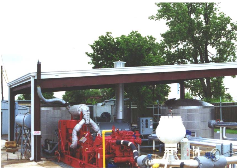
Fig. 3.18 Canopy cover over the boiler
