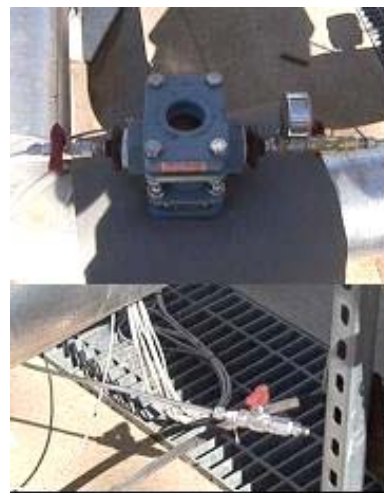
Fig. 7.3 Removable view port and bottom sample port
