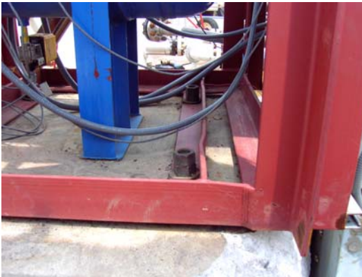
Fig. 3.59 Deformed mast support structure
